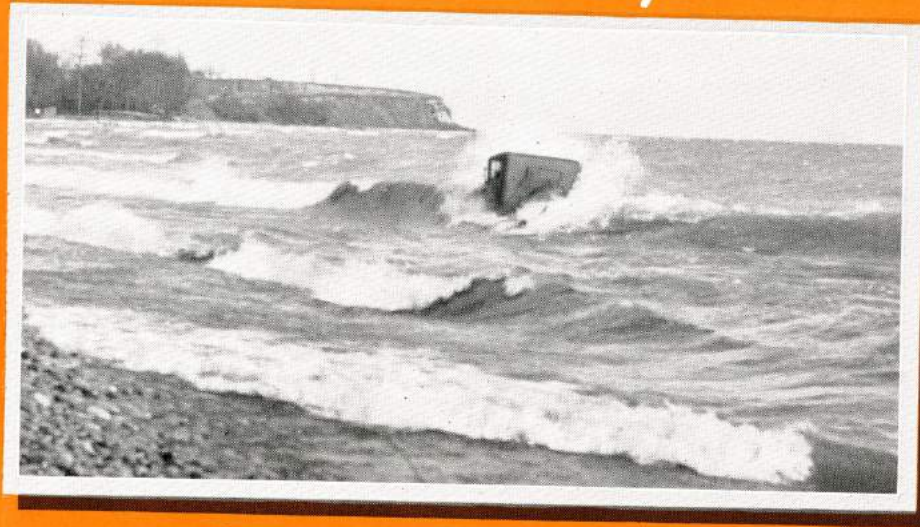
Waterproofing Test, Lake Ontario
