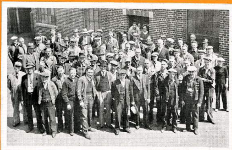
Heavy Reject Men, Oshawa 1944
