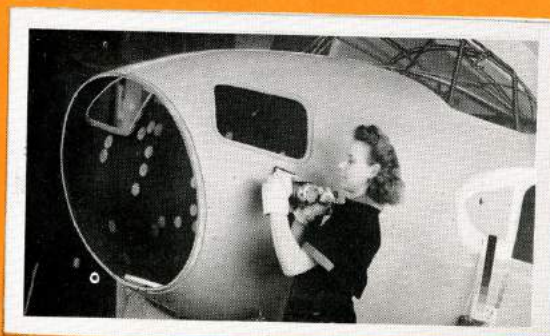
Smoothing the Surface
