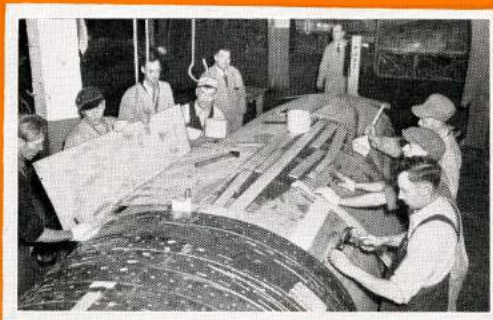
Plywood Skin Goes On
