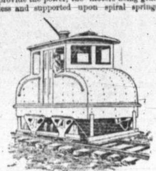
HIGH SPEED ELECTRIC LOCOMOTIVE. having their base on the side frames of the truck. This arrangement gives the wheels a certain freedom of movement irrespective and diminishing the wear and tear upon | hazardous for Coleman to try it again. the tracks and the motors.
