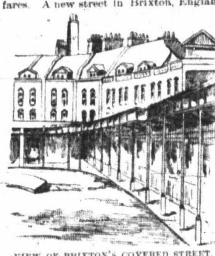
covered pavement on each side is ten feet wide. Light fron pillars support a glazed roof, from which are suspended numerous he same time thoroughly protected from storms and heat.
