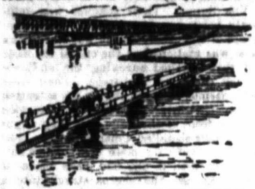
PONTOON BRIDGE AT NEBRASKA CITY. be impracticable. However, the bridge has been built, and it is said to be the largest pontoon bridge in the world. The especial feature is a V shaped draw, with the angle of the V down stream, which the current may open whenever required. The draw is so constructed as to be closed by one man.
