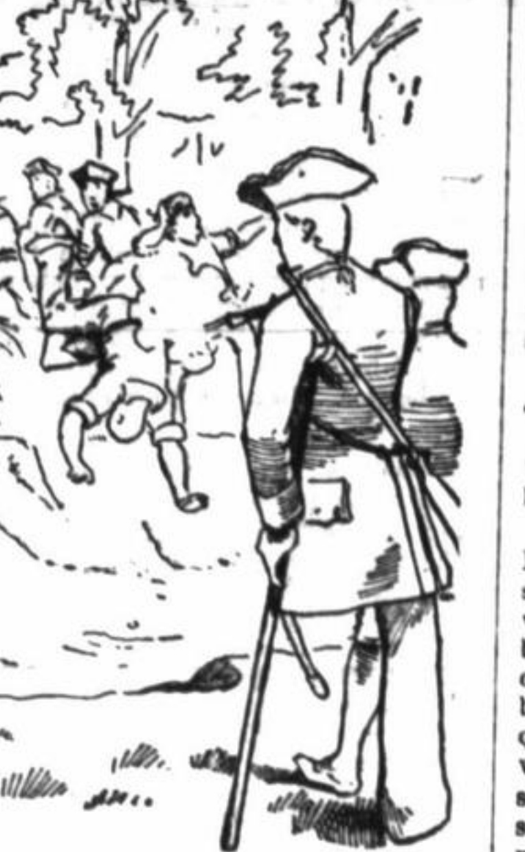
Merry tumbled head foremost into the excavation.
