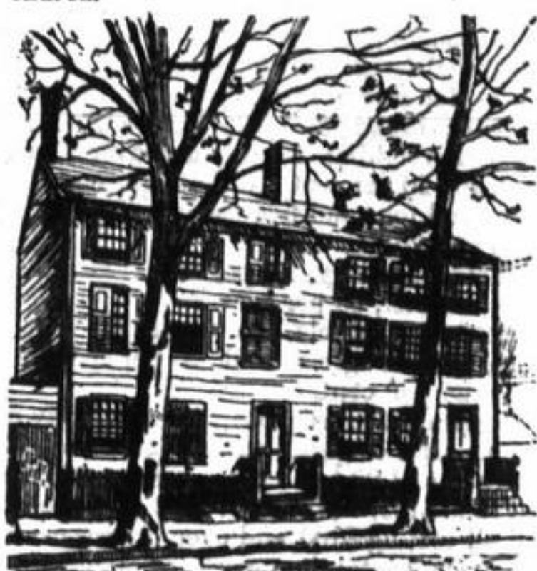
144 AND 146 ADAMS STREET, BROOKLYN. Building in which first Sunday school in Brooklyn was held.
