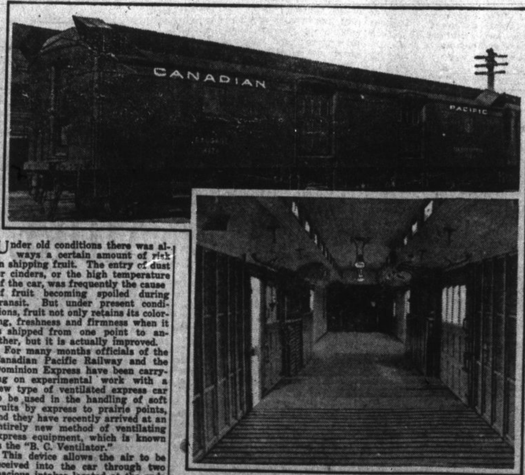
New type of fruit car showing special ventilators, on the top of the car, which aid the fruit to retain its freshness. Lower picture shows interior of the modern fruit car.
