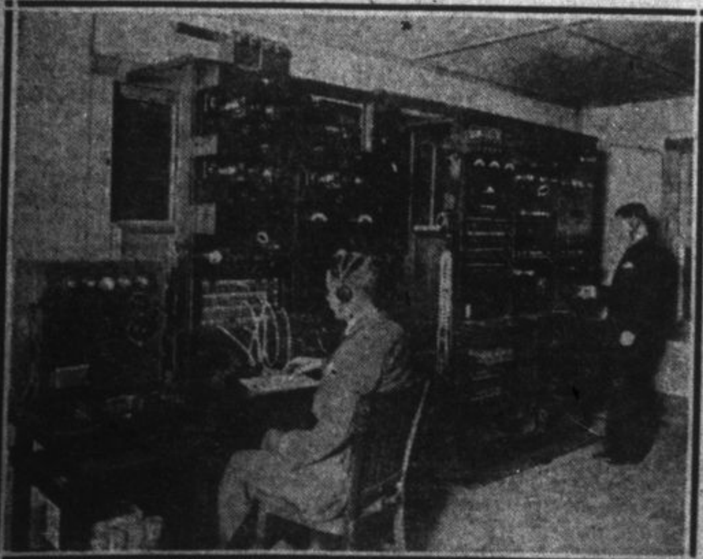
INTERIOR OF RADIO RECEIVING STATION.
