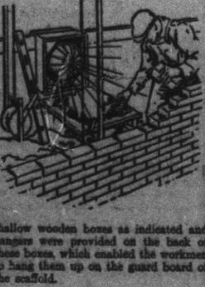
Shallow wooden boxes as indicated and lamps were provided on the back of these boxes, which enabled the workmen to hang them up on the guard board of the scaffold.
