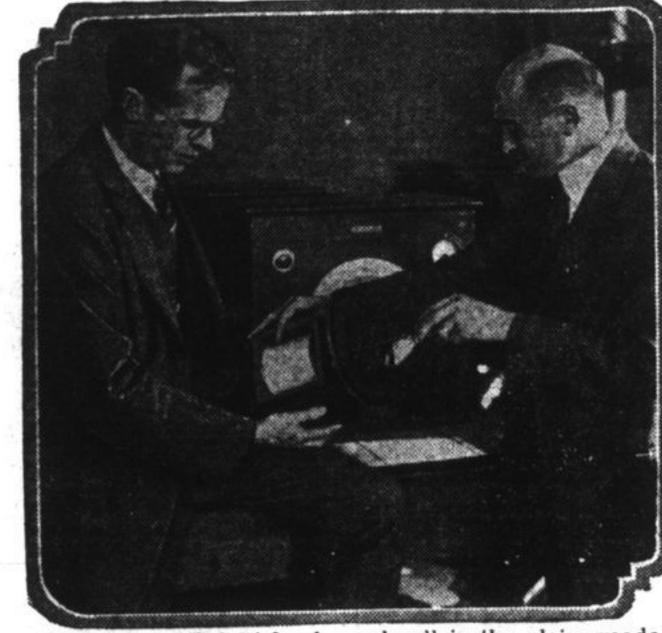
"The most efficient loud speaker." is the claim made for this new appliance designed by Chester W. Rice and Edward W. Kellogg at the General Electric laboratories in Schenectady, N.Y. The unit contains an amplifier, besides a new type of loud speaker, all of which works from house current. Kellogg, at left, and Rice are shown adjusting the loud speaker with the rest of the unit behind them.
