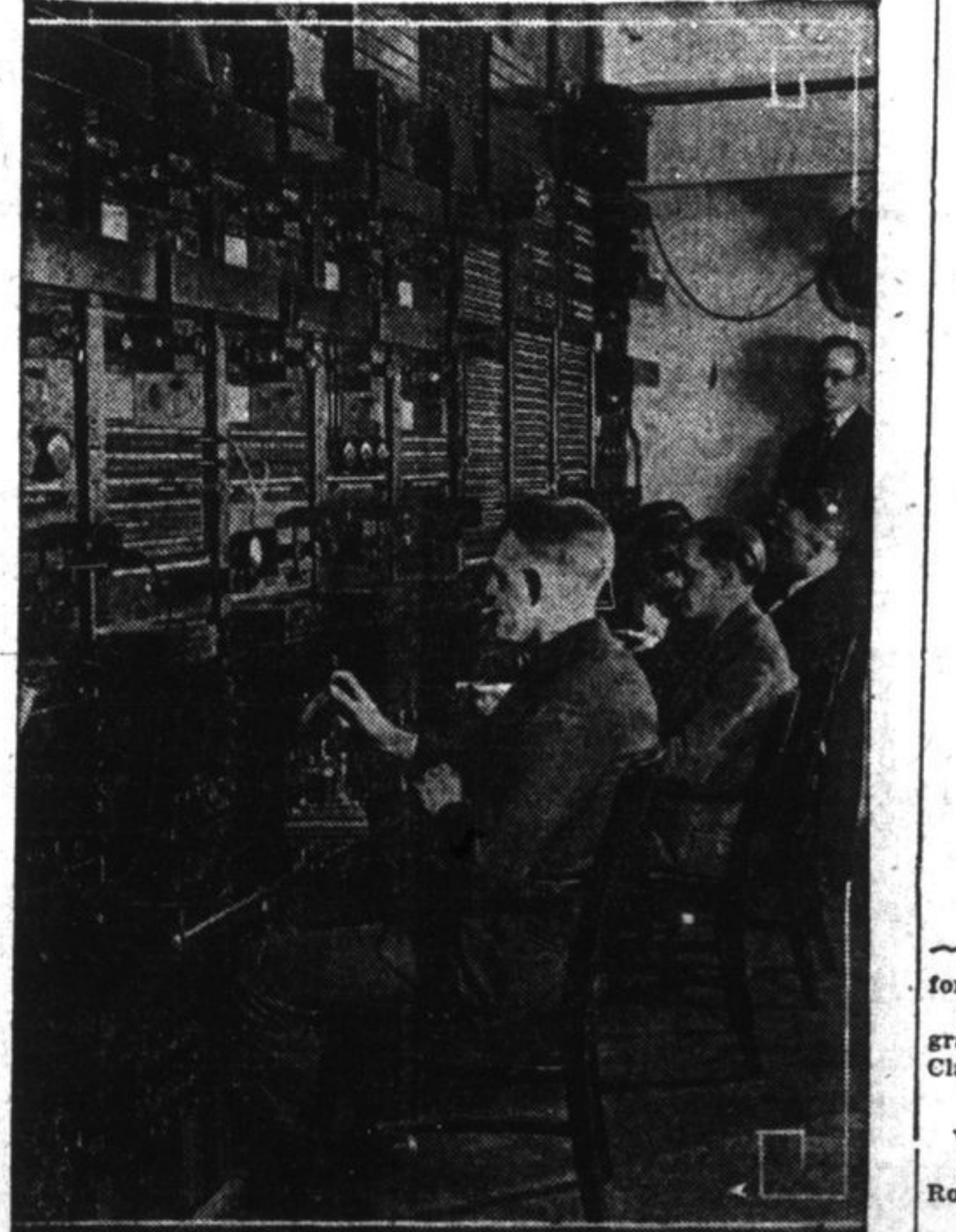
The "Switchboard" of WCAP, at present the world's greatest broadcaster. Through this panel go the lines connecting 13 other broadcasters.
