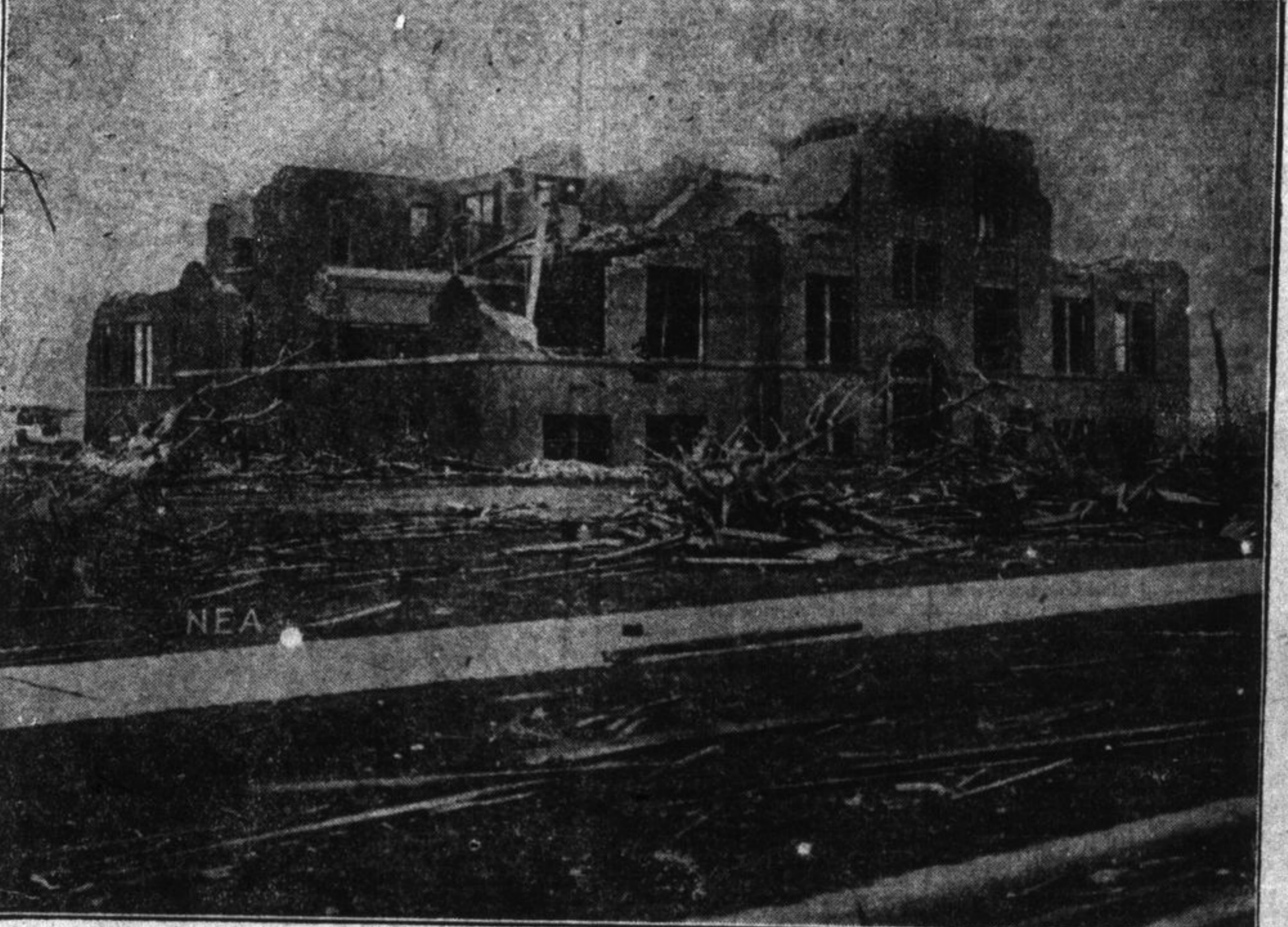
Ruins of the Longfellow grade school at Murphysboro, Ill., where approximately seventy children were crushed to death when a tornado of unprecedented fury swept through the town, snatched off the roof of the building and piled the dead and injured in heaps.
