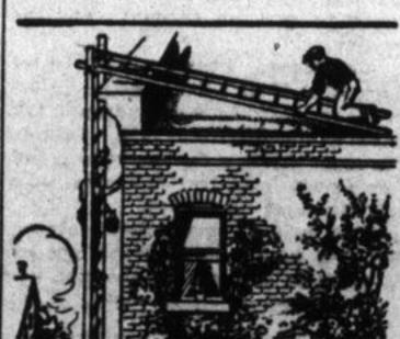
climbs down the vertical ladder, the arrangement in position. The horizontal ladder should not project over the edge of the roof more than one-fourth or one-fift! the entire length of this ladder and the man holding it down must apply his weight at the extreme inner end; he mus be about equal to the other man in weight
