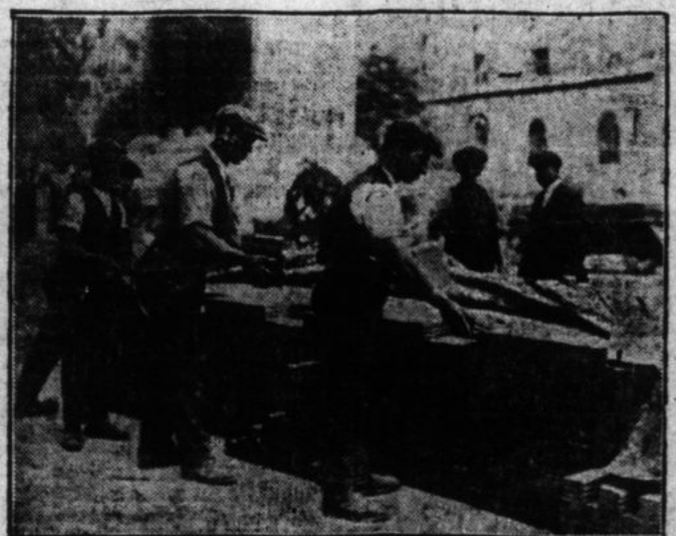
SILENCE AT THE EMPIRE'S CENOTAPH. The pavement around the famous Cenotaph in Whitehall, London, is being replaced with rubber to deaden the sound of traffic. The workmen are seen unloading the rubber blocks.
