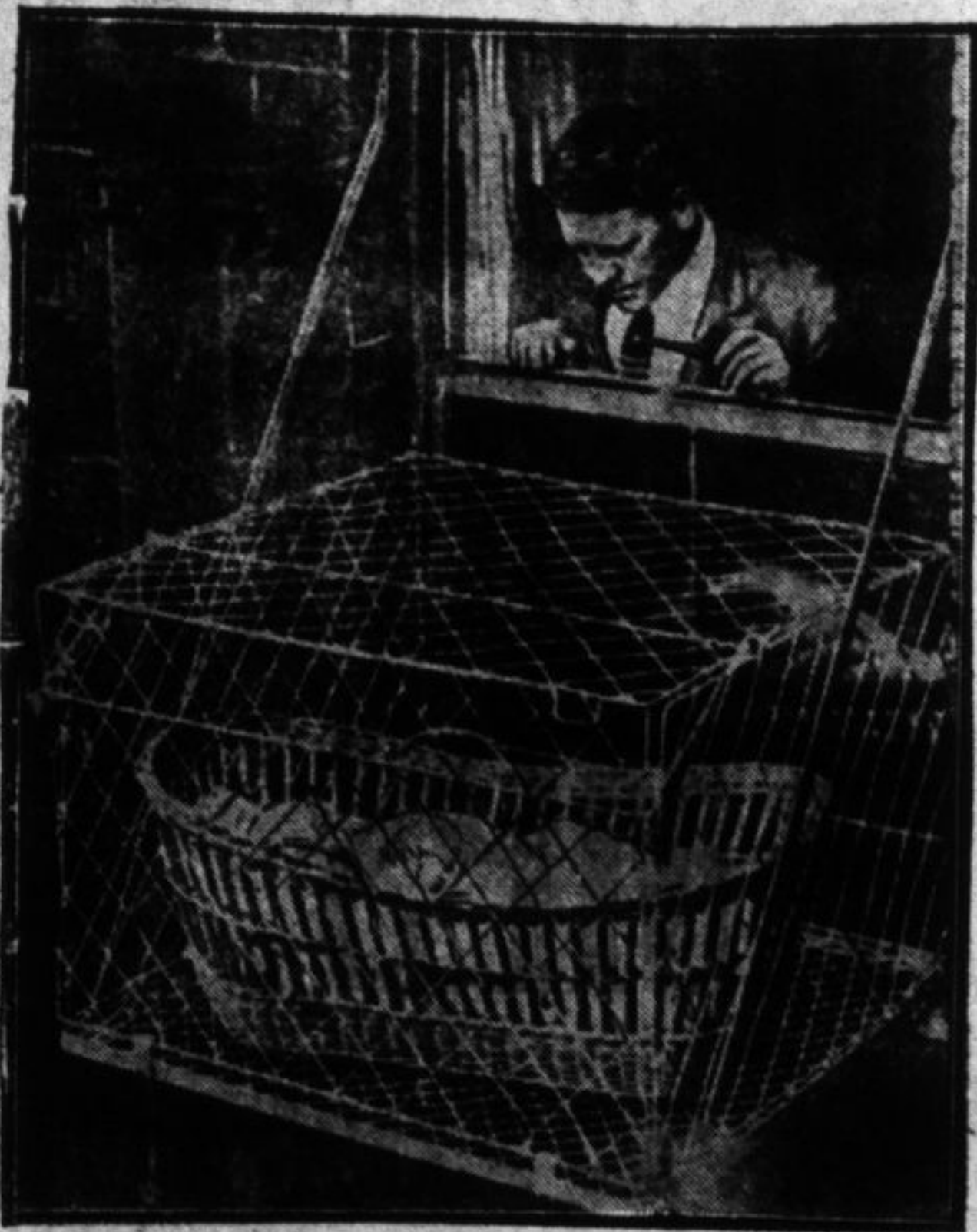
This father has solved the dark and poorly ventilated flat problem by building a cage outside his third-storey window for his baby.
