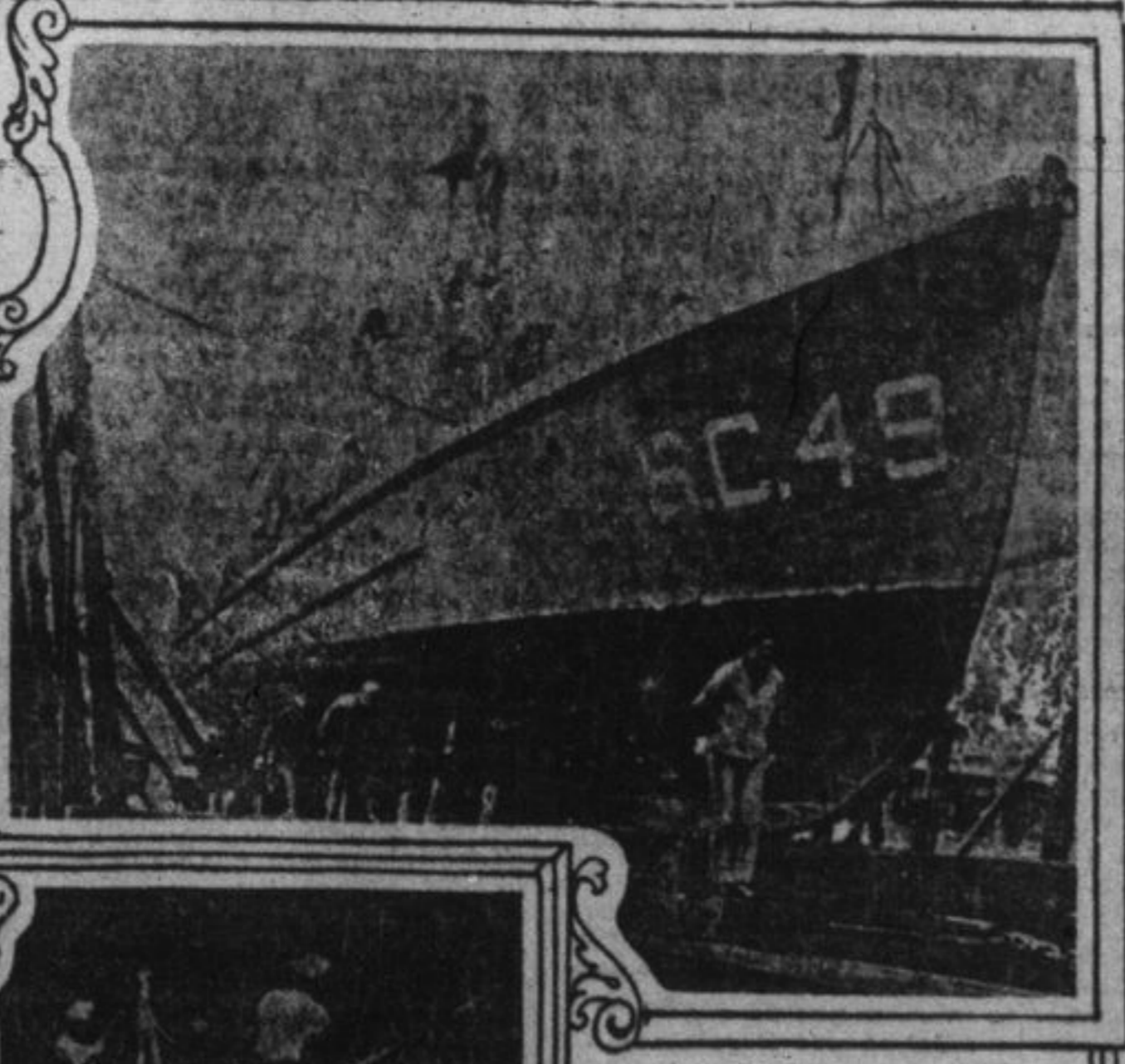
LAUNCHING A SUBCHASER In Brooklyn Navy Yard the big traveling crane came up and lifted these motor boats from the ways and lowered them into the water.
