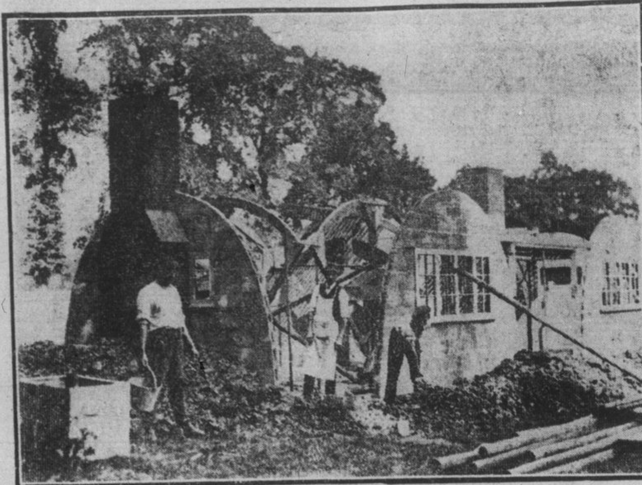
England is greatly interested in a new method of building concrete houses, which is being demonstrated by Maurice S. R. Adams, F.R.I.D. The house shown in the picture would be built in a fortnight's time.
