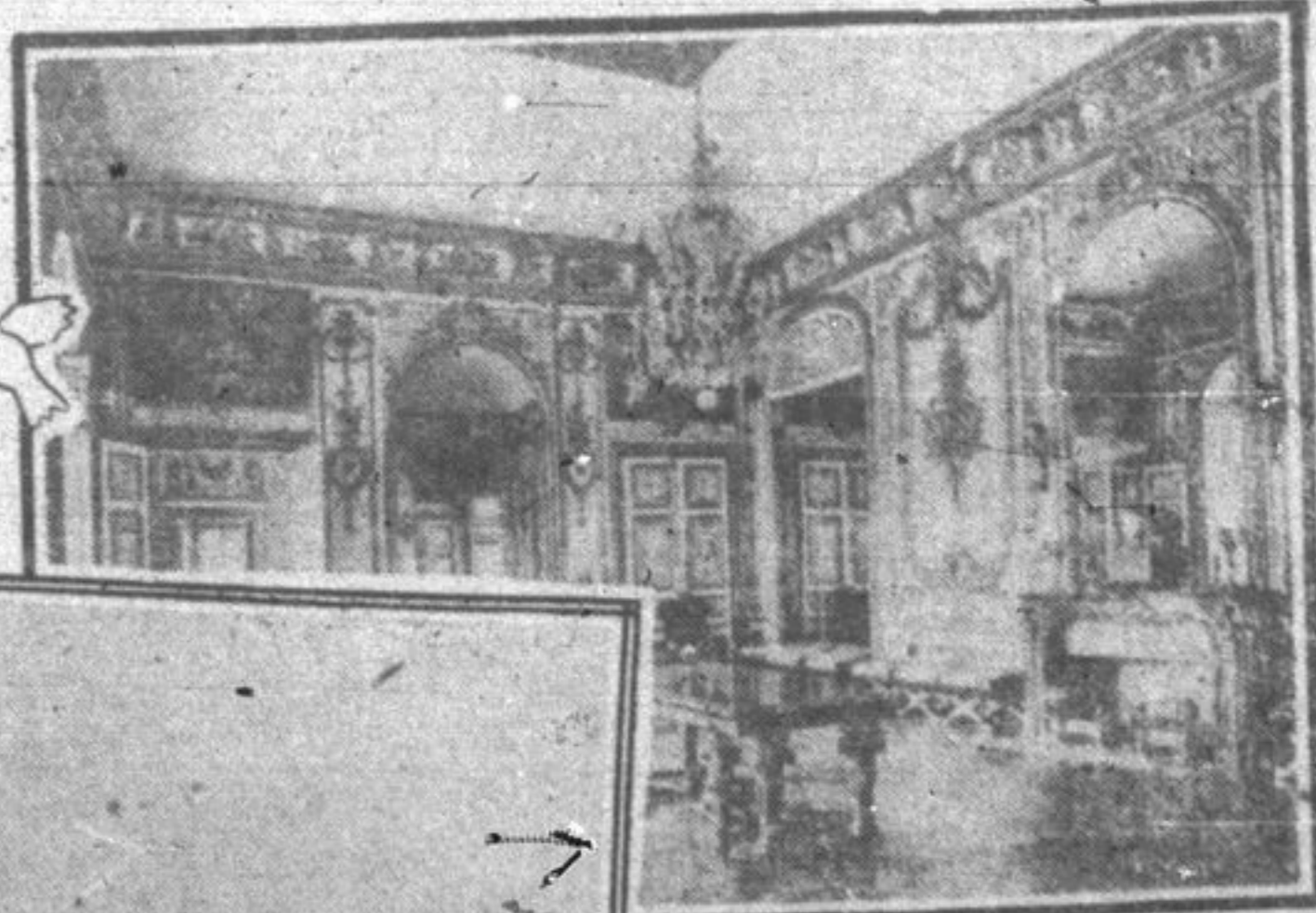
One of the Council Rooms
