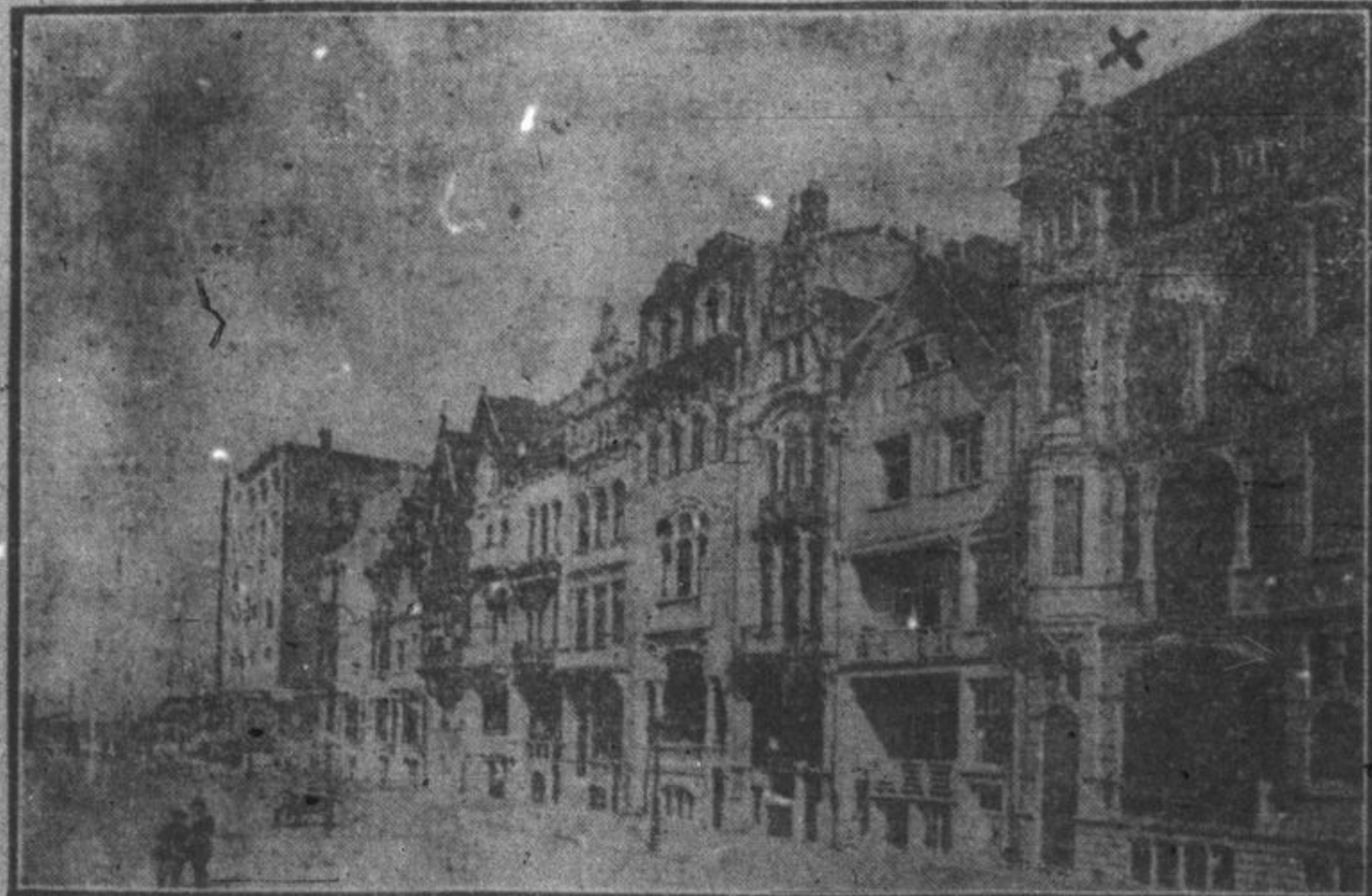
THE DIGUE AT MIDDLEKERKE.
