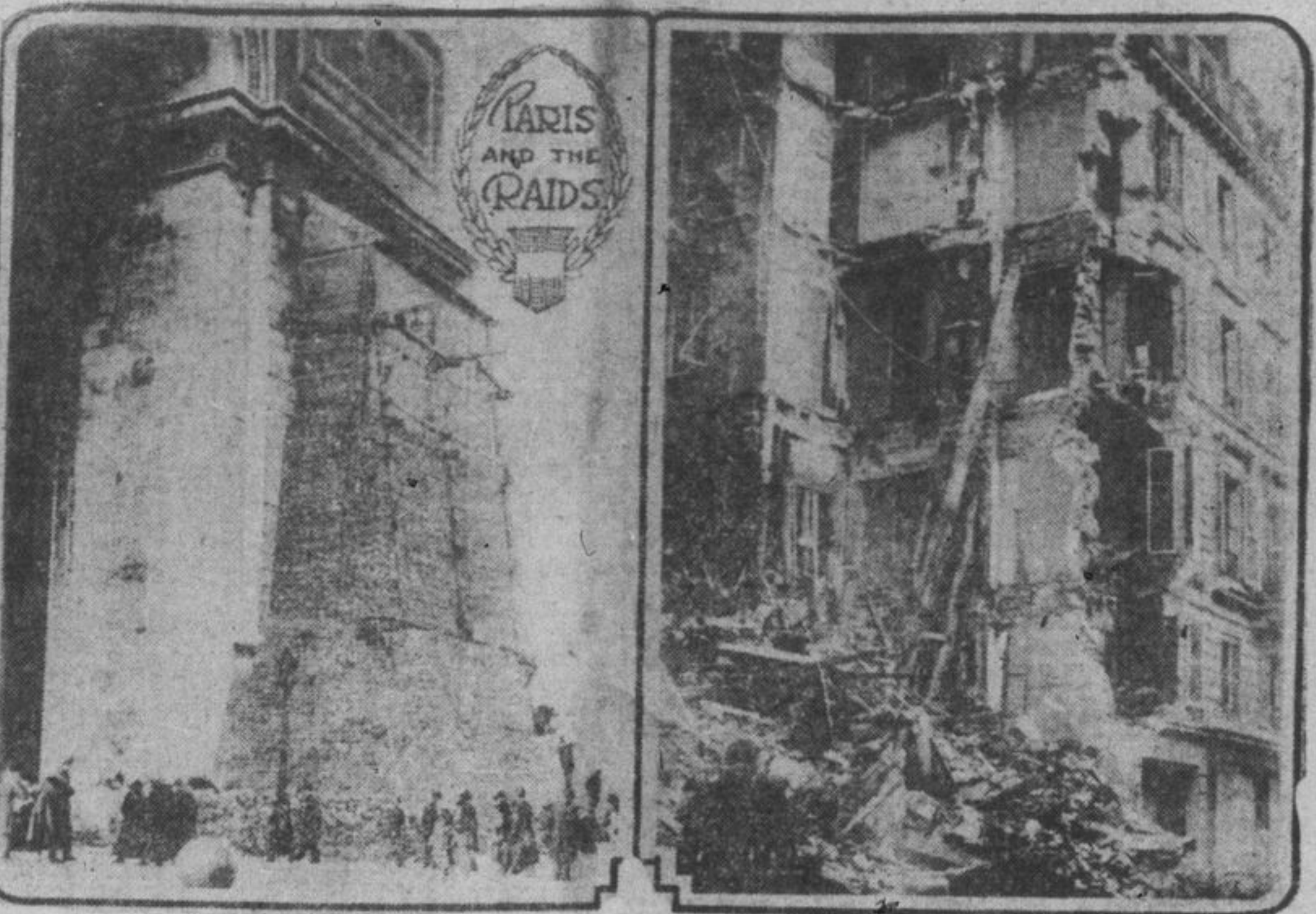
The left hand picture above shows the Arc de Triomphe protected by sand bags to preserve from bombs and shells the famous sculptures which adorn it. The arch was begun by Napoleon I, to commemorate his victories, and the sculptures are in large relief on each of the four sides of the facade near the base. The right hand picture shows the damage wrought by a single bomb on a typical six story apartment house in Paris. Two hundred persons took shelter in the cellar of this building, despite the destruction of the upper floors, and all were taken out safely after many hours.
