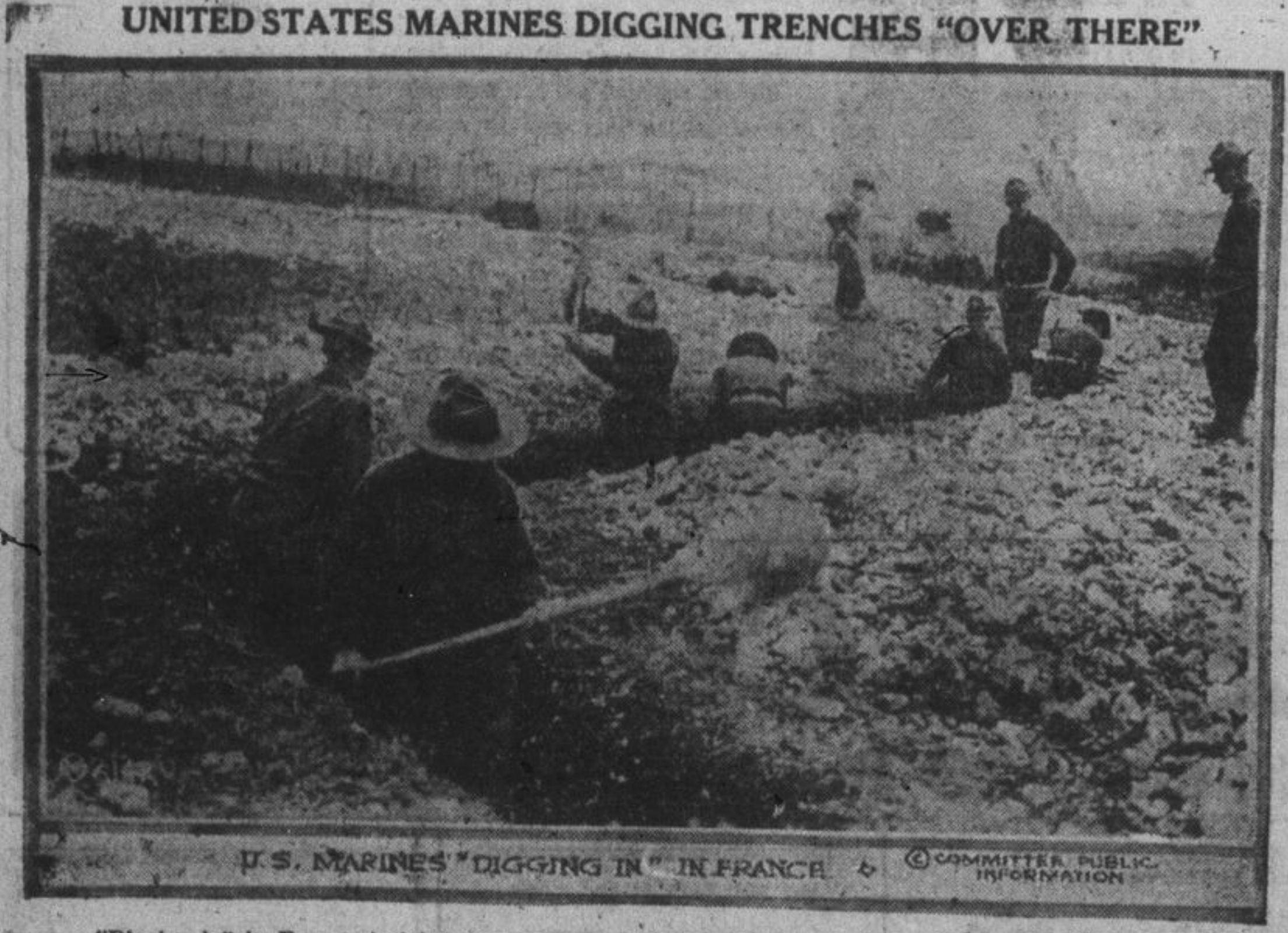
U.S. MARINES "DIGGING IN" IN FRANCE
