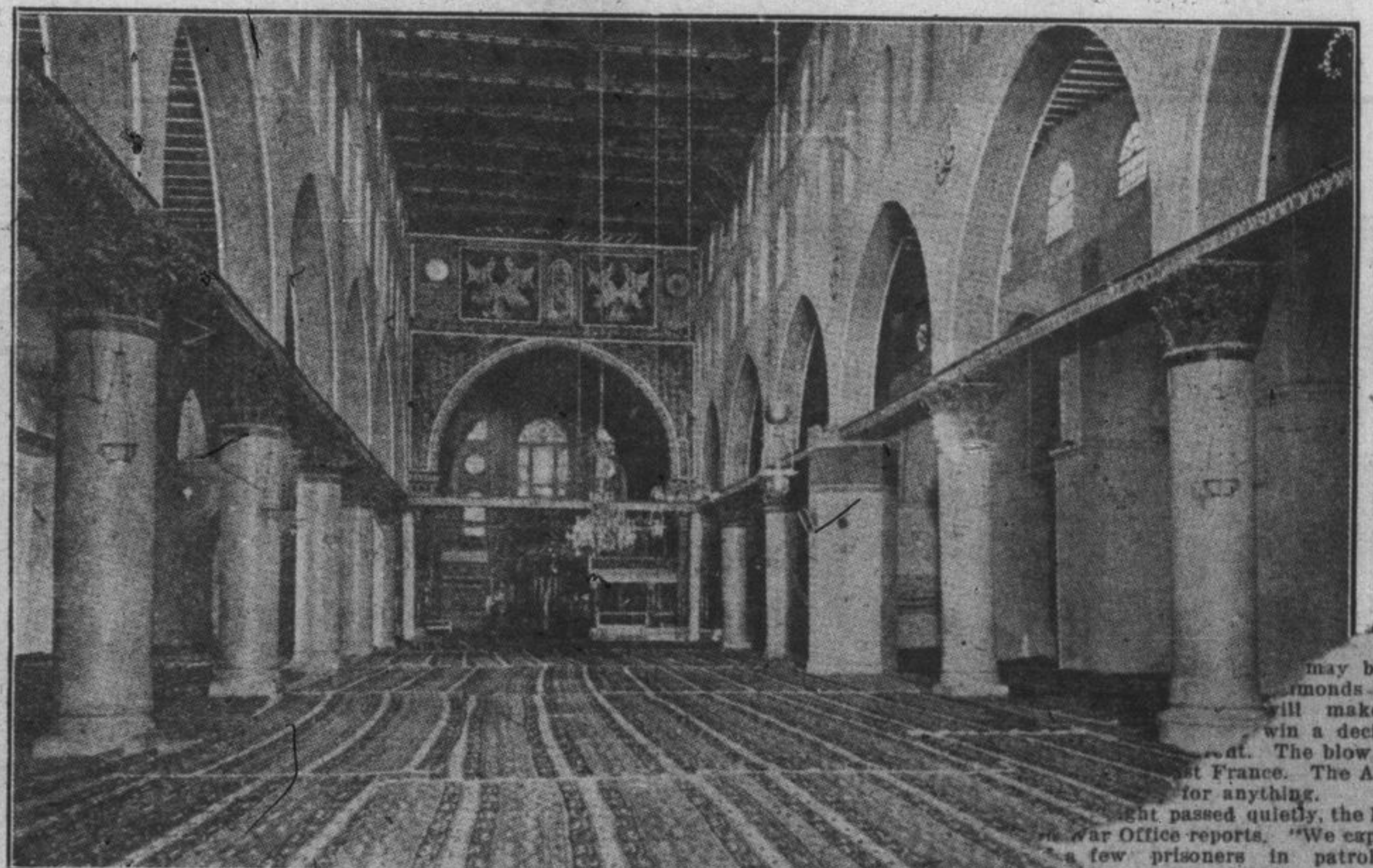
The interior of the Mosque El-Aksa in Jerusalem. The magnificent basilica, built by Justinian in 530, was converted into a mosque, but some traces still remain of the original building. The porch still contains two niches for statues, the work of the Templars.
