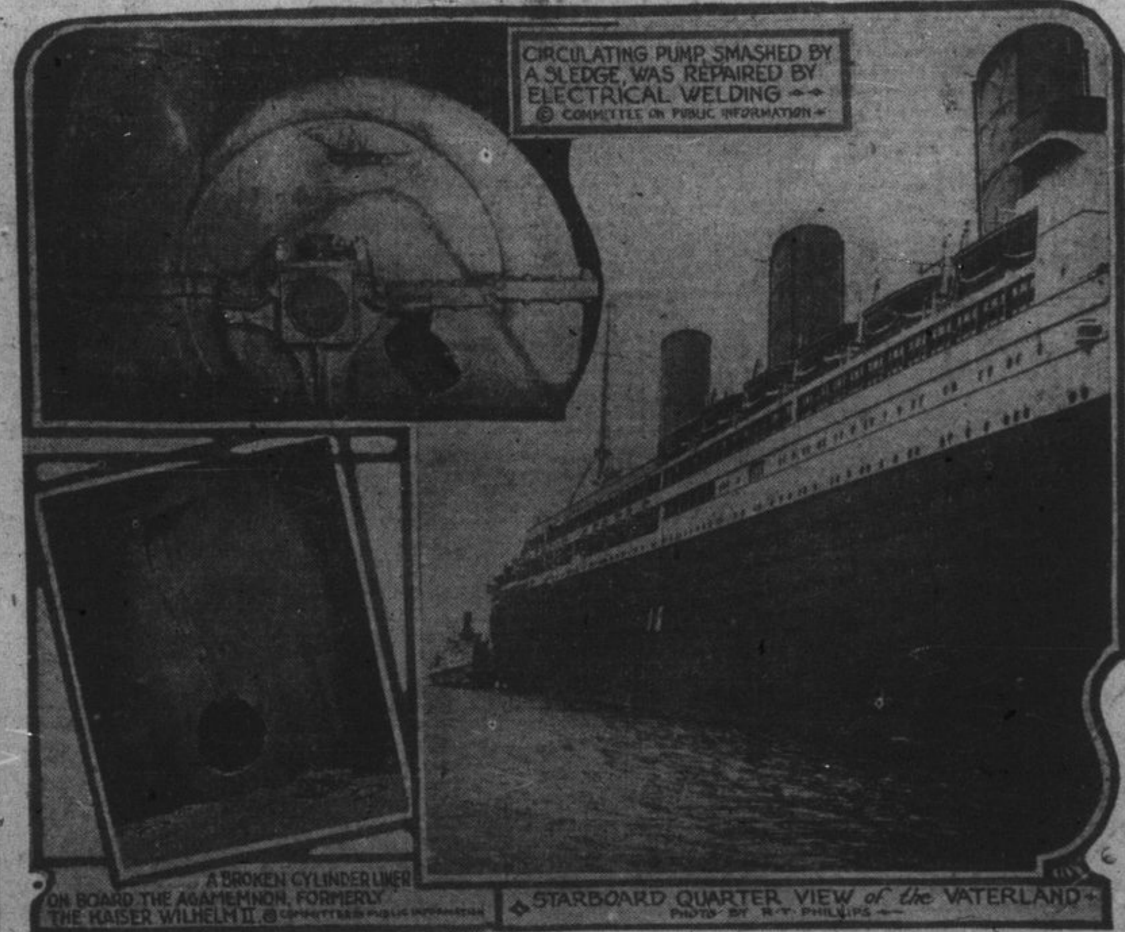
One of the photos shows the Vaterland starting on one of her latest trips. Another photo shows a broken cylinder liner on the U. S. S. Agamemnon, formerly the Kaiser Wilhelm II. The photograph shows how the liner was split and the beginning of the process of repair through welding. The third photo is typical of the vandalism found on all of the German ships. With a battering ram or a sledge the vandals smashed this circulating pump casing. It was repaired by the electric welding process, and the ship is in active service to-day.
