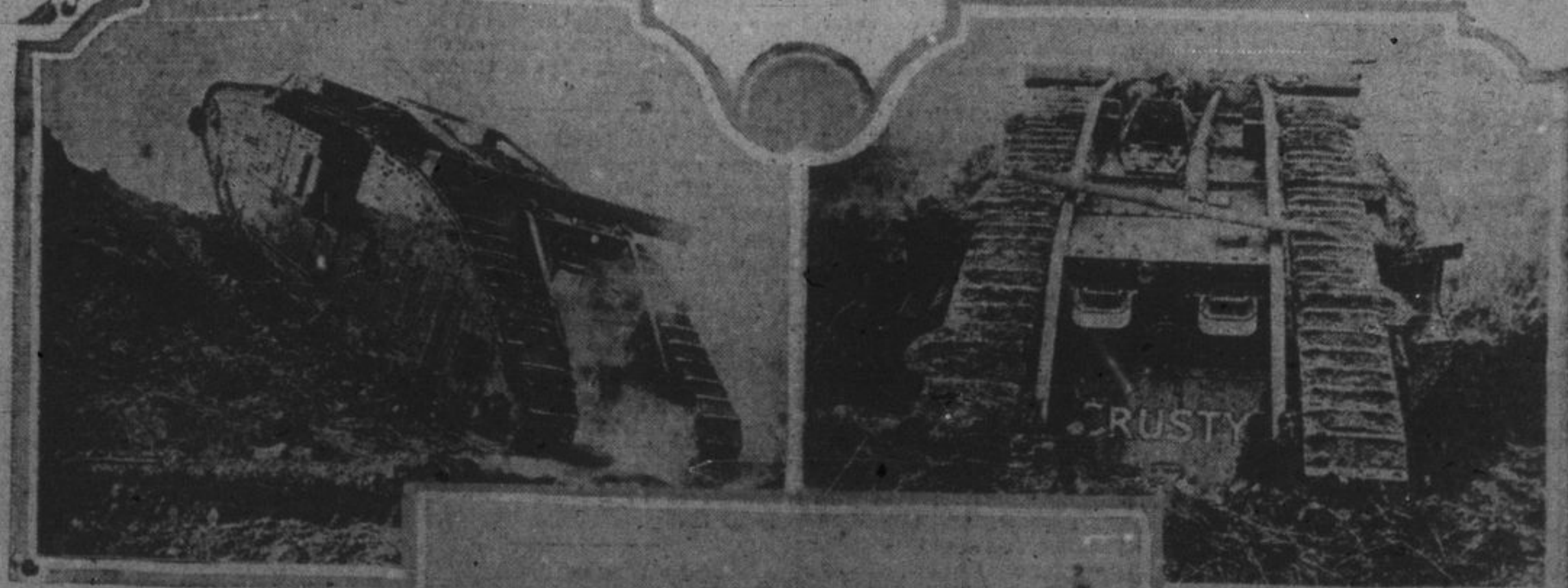
The upper left shows the tank creeping on a slope leading downward into a ditch. Fumes are issuing from one end. A heavy bar is visible above the rails in close proximity to the big links above the body of the tank. The upper right photograph shows the forward portion of No. 5 lying on soft ground. The travelling links are loaded with soft earth.
