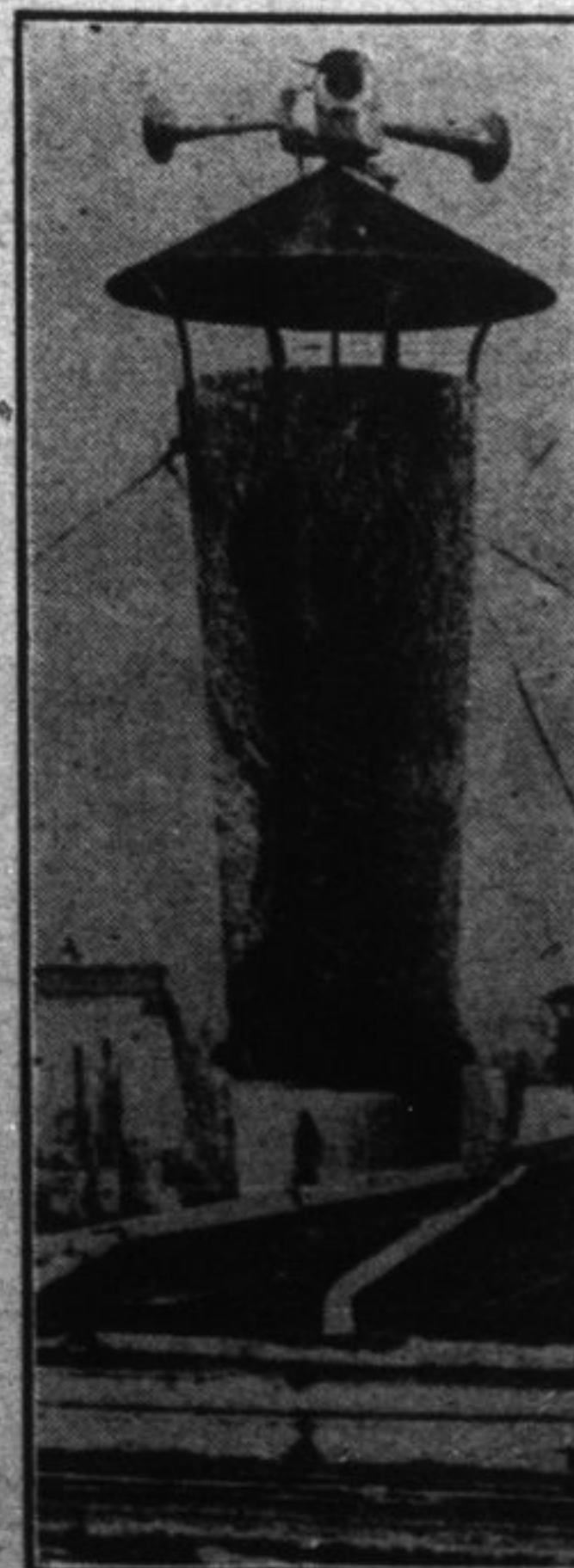
One of the many sirens on Paris roofs which give warning of the approach of enemy aircraft.
