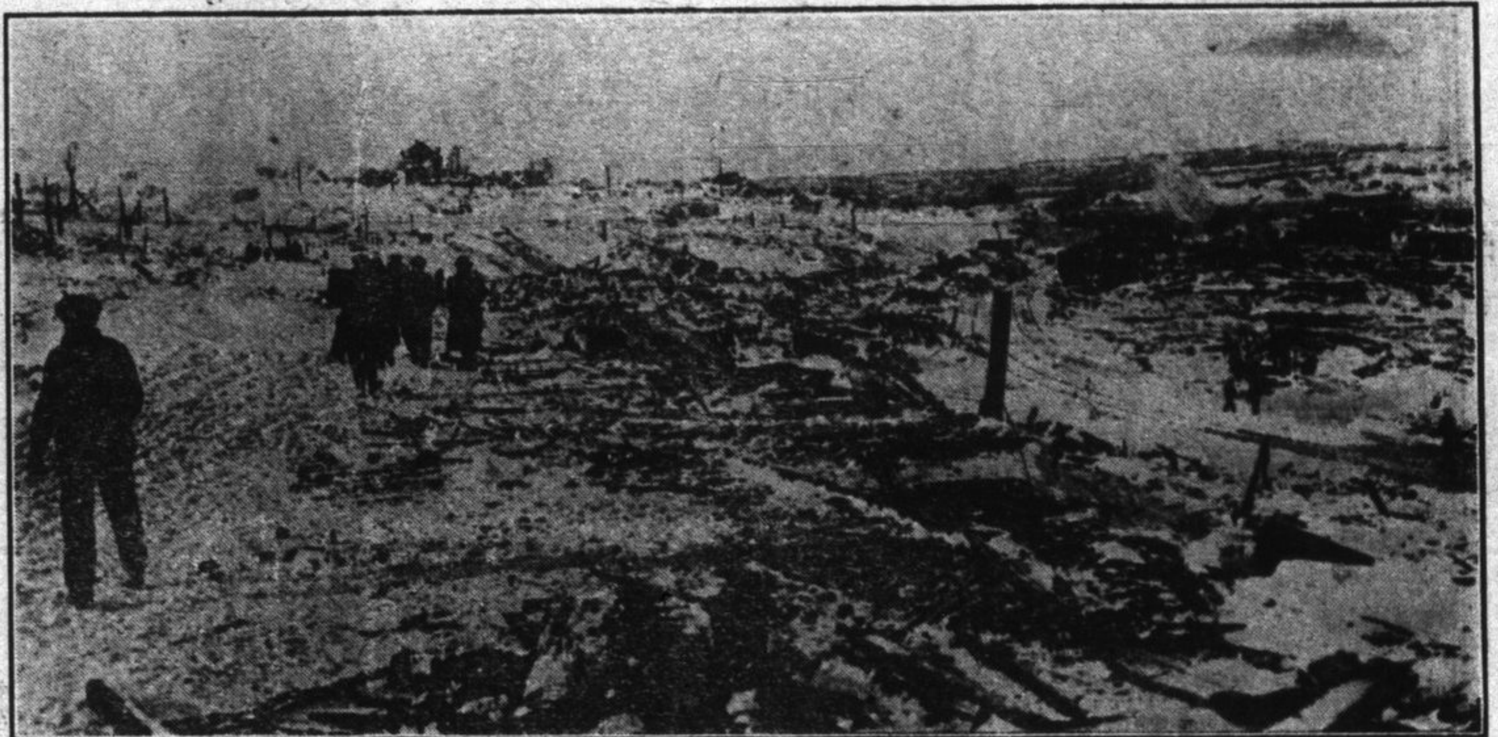
General view of the wrecked city of Halifax along Barrington Street, one of the most populous thoroughfares. In the area shown hundreds of houses were shaken down and the debris was consumed by fires. Scores of human beings perished here, and a blizzard that followed made the rescue work almost impossible for several days. Few persons survived the explosion at this spot, close to the waterfront.
