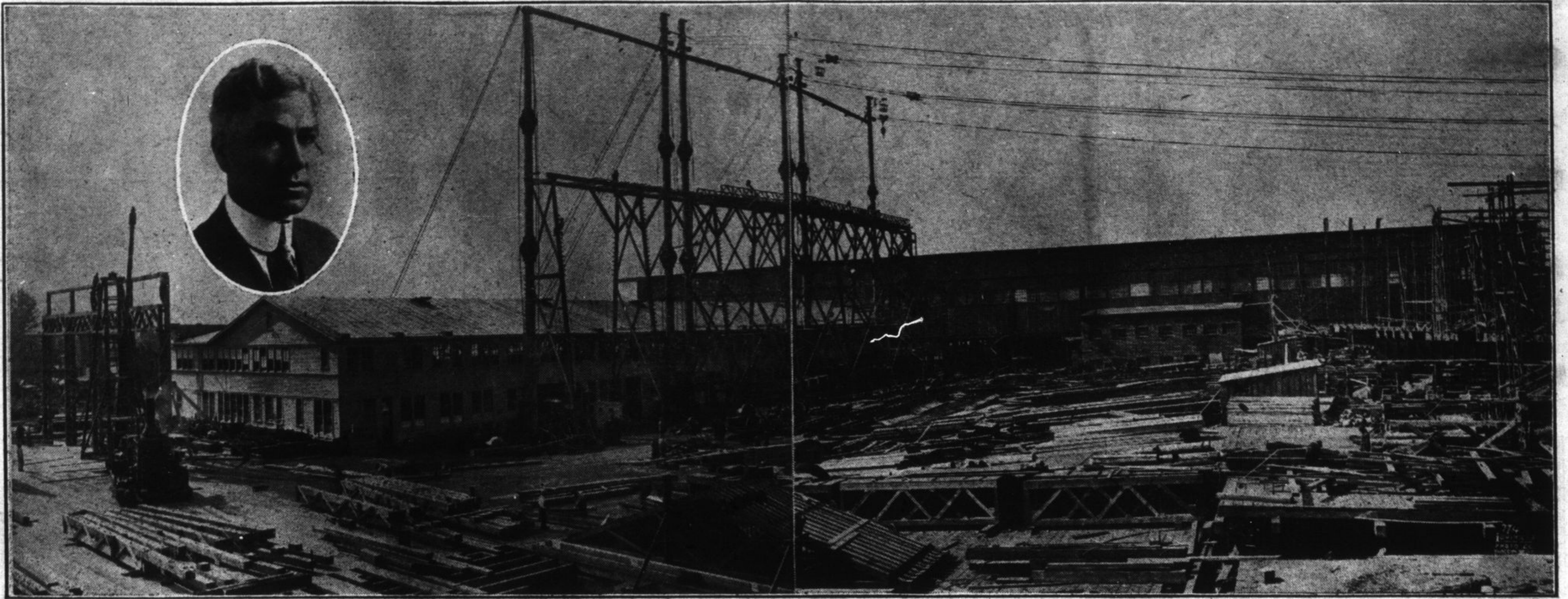
A splendid panoramic view of Coughlan & Sons' steel shipbuilding yards at Vancouver. The man in the insert is Mr. J. J. Coughlan, Jr., managing partner of this firm.
