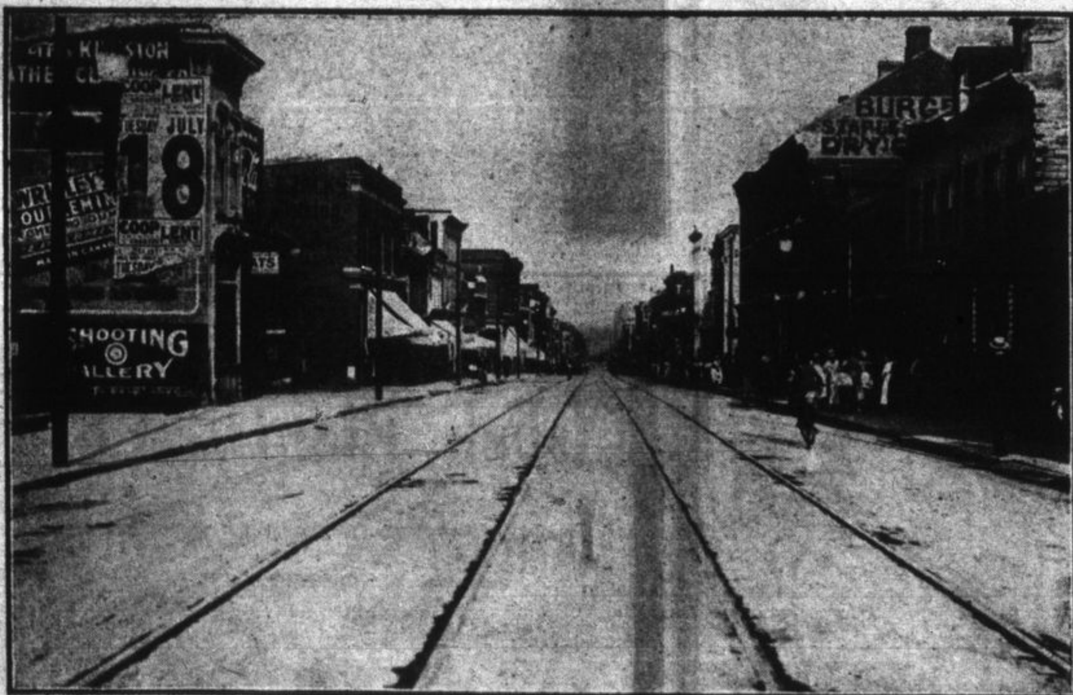
Looking down Princess Street from its junction with Clergy Street. This street was paved in 1914 with asphaltic concrete, with sandstone blocks in the track allowance.
