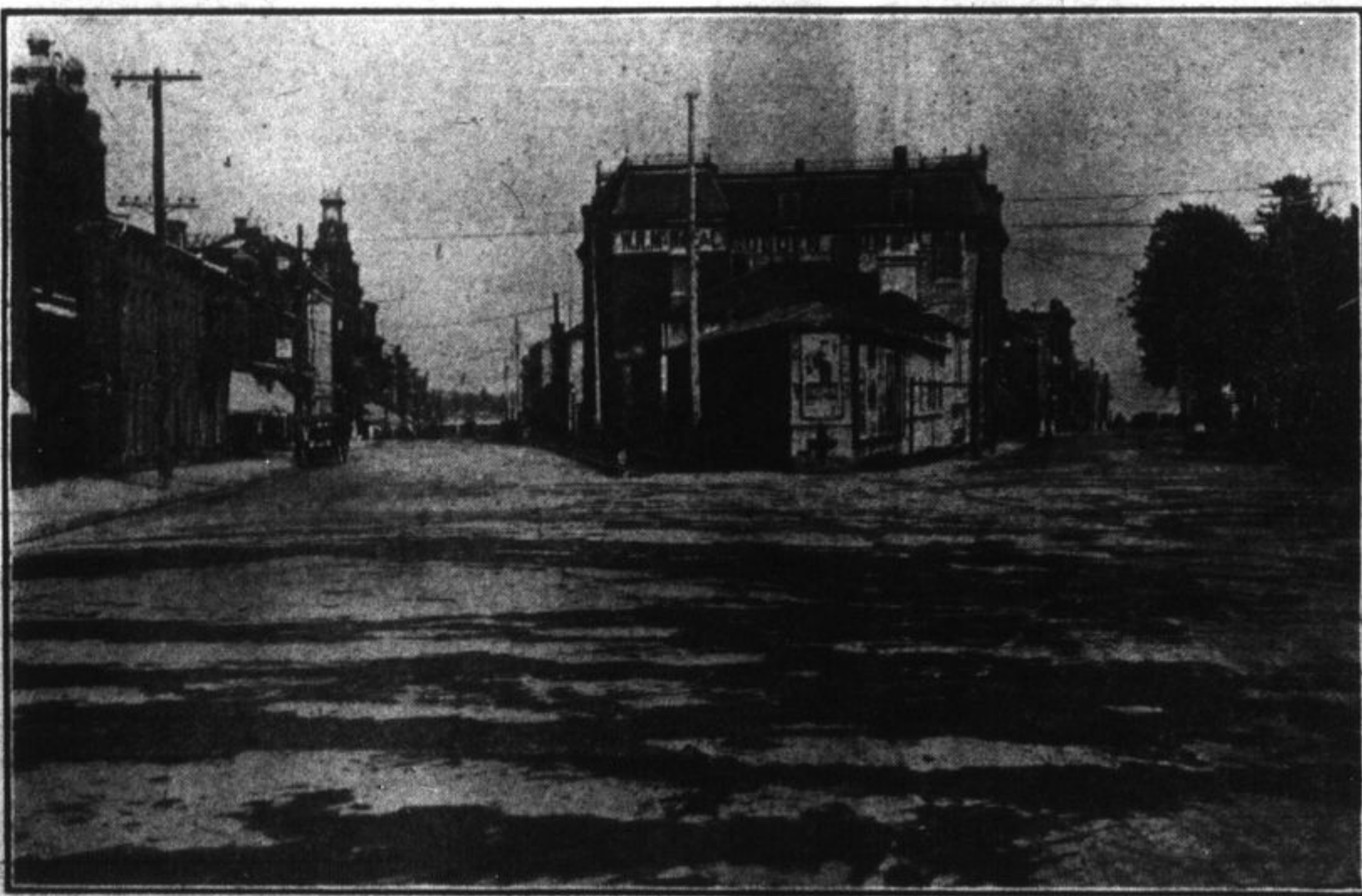
Junction of Brock and Clarence Streets, showing the Golden Lion Block in the centre. This section was paved with asphalt block in 1912.
