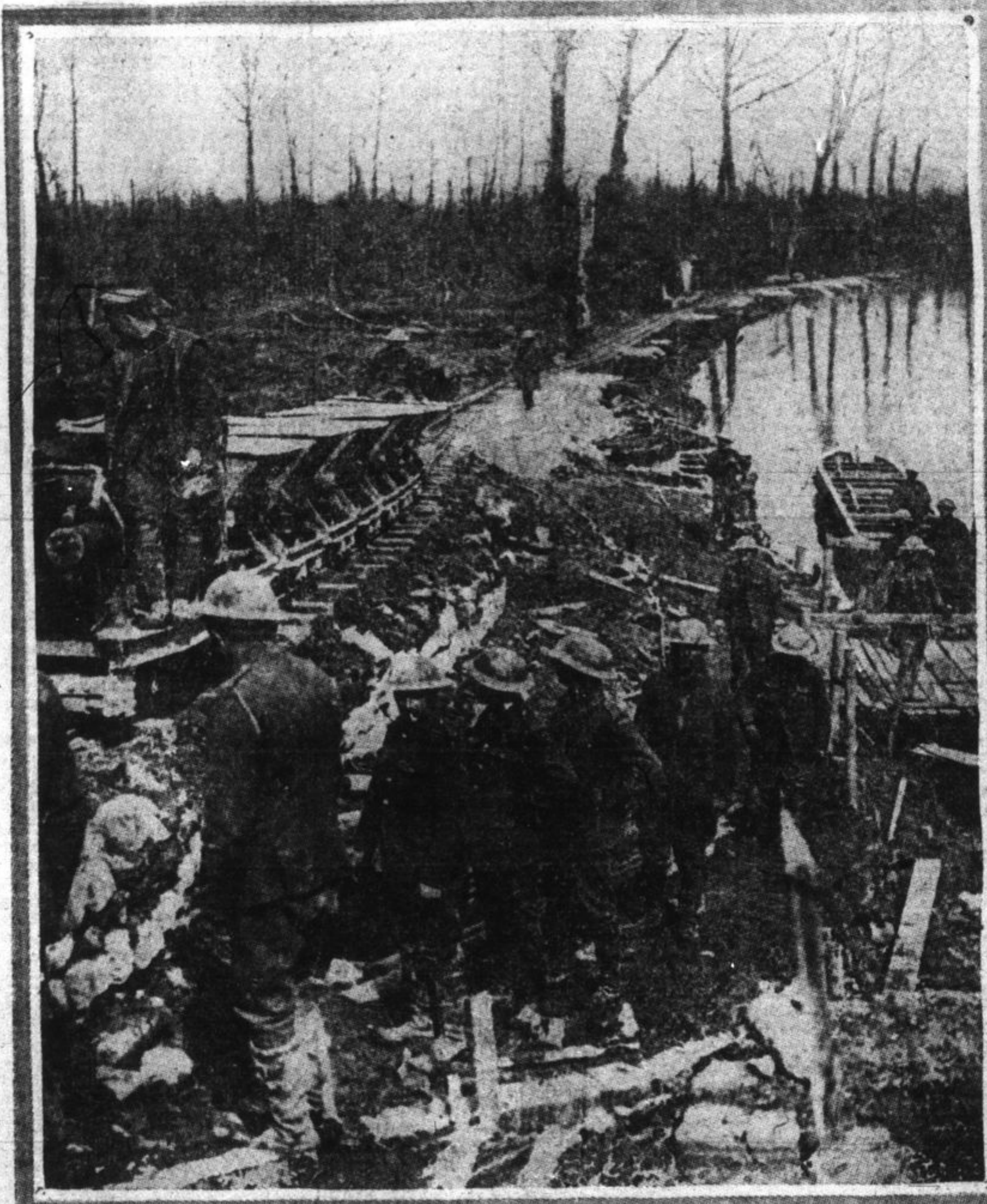
The accompanying picture shows the arrival of a truckload of shells at the point where they are to be transferred to pontoon boats for transport nearer to the front. The light railways have proved themselves to be invaluable in modern warfare and follow the line of advance very closely. The pontoon boat, built by British engineers, is moored close to the bank and a party of gunners are returning to the railway, which here runs alongside a canal, for a further load of shells. The next stage is the journey of the shells from the base to the positions where the guns are waiting for them.
