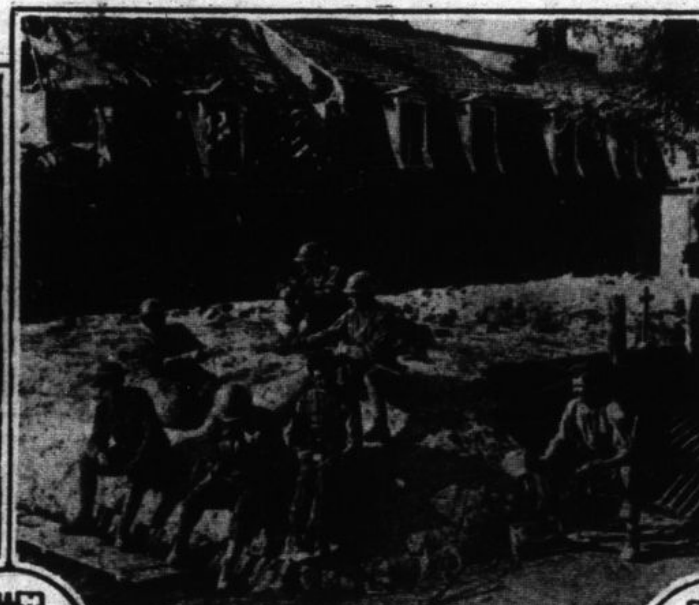
Canadians at home in a concrete fortification made by the Germans in a French village.
