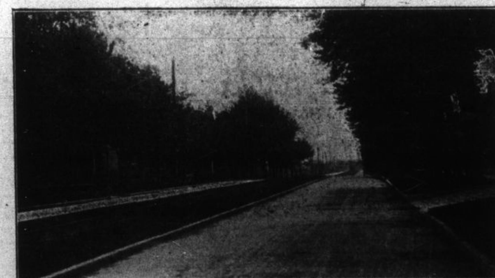
WILSON AVENUE, ST. THOMAS. Two concrete pavements 18 feet wide and 7 inches thick, laid in 1913. The track allowance is 20 feet wide. The sidewalks are 5 feet wide and the grass spaces next to the curbs are 12 feet wide. The width between property lines is 100 feet.
