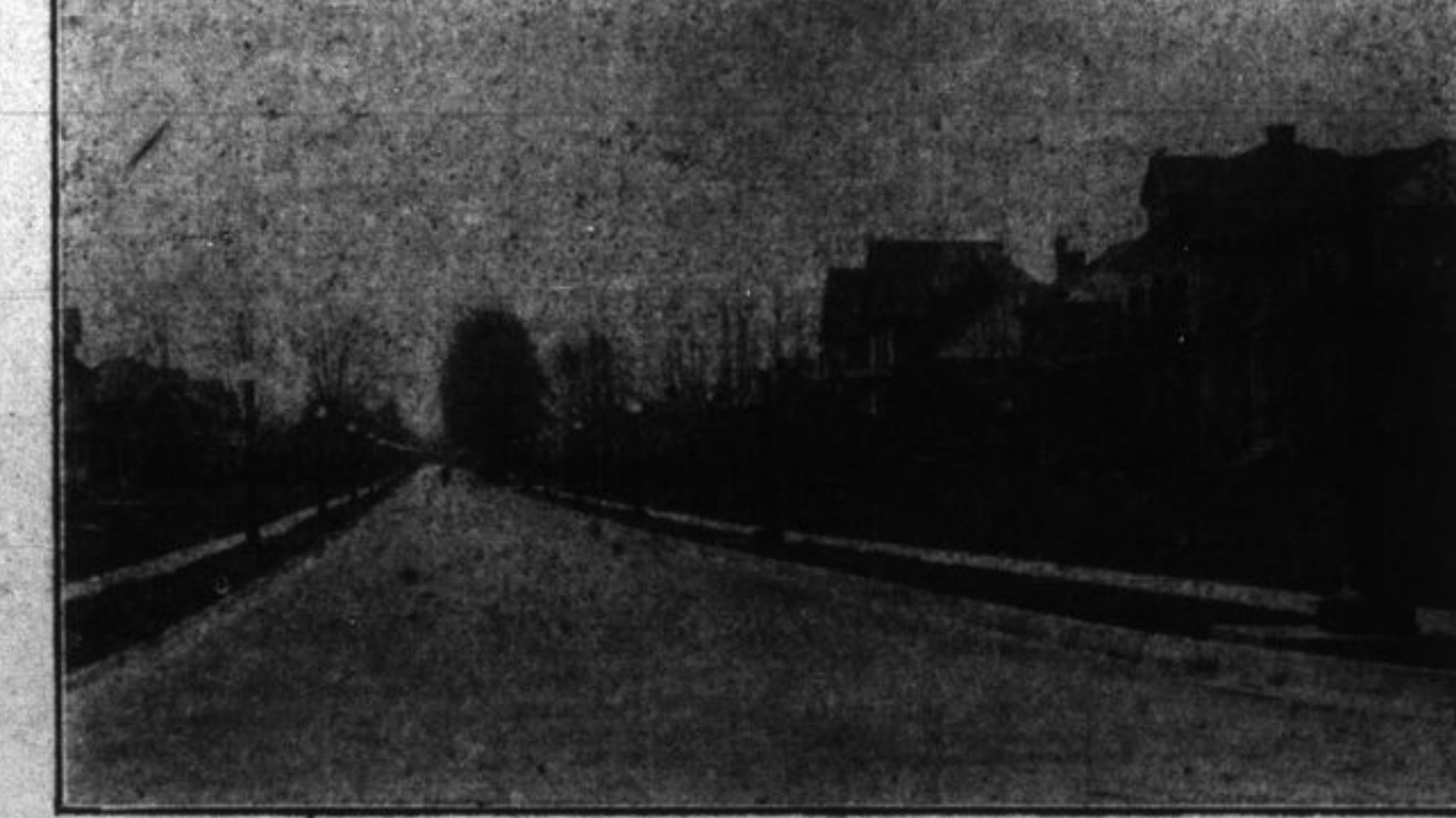
BRANT ROAD, GALT. Tar filled macadam surface 26 feet wide on a broken stone foundation, laid in 1911. The sidewalks are 5 feet wide and the grass spaces next to the curbs are 3 feet wide.
