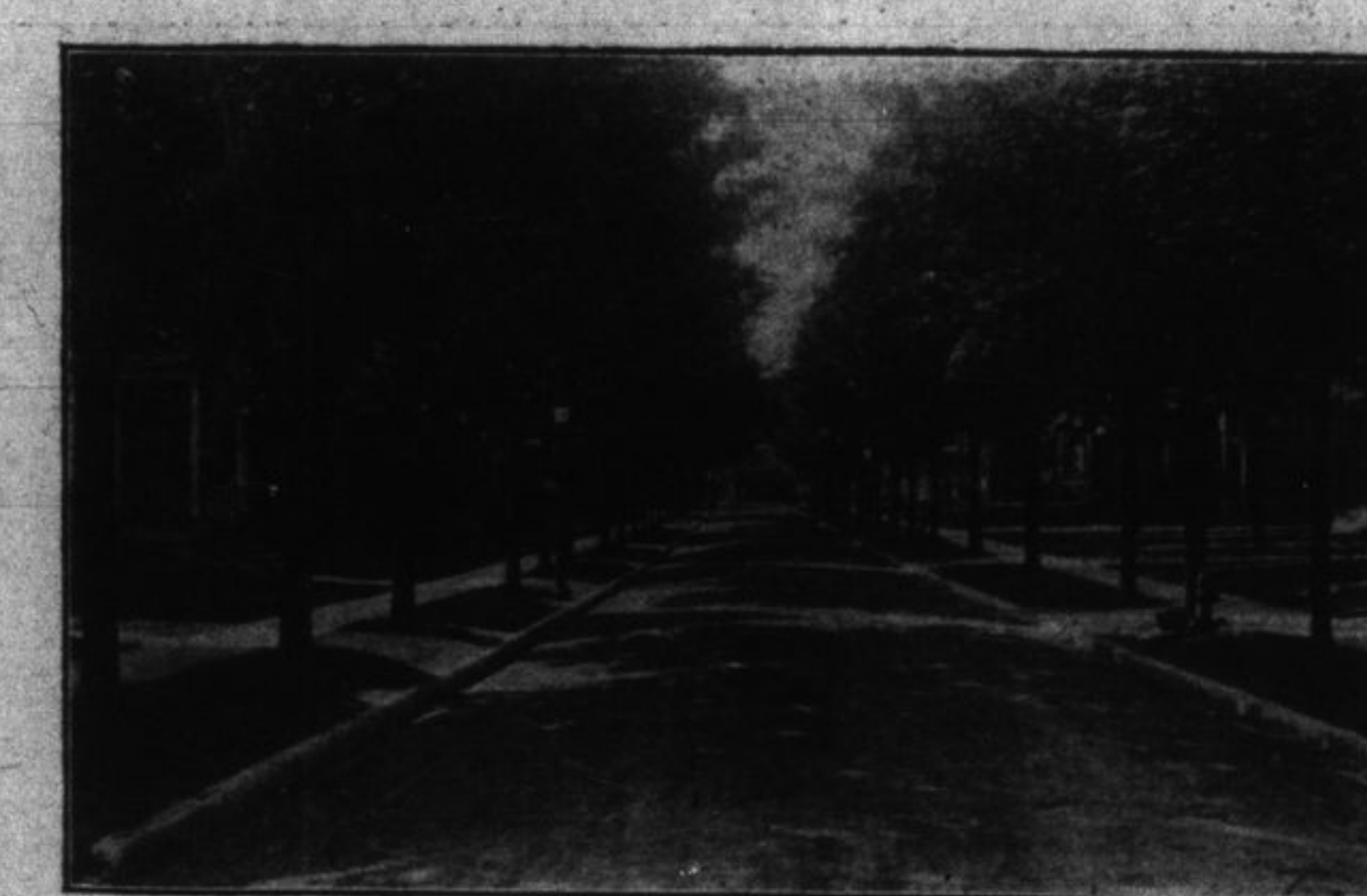
PARK AVENUE, GUELPH. Water-bound macadam roadway, with surface application of cold tar, 22 feet wide, laid in 1915. The sidewalks are 5 feet wide and the grass spaces next to the curbs are 7 feet wide.
