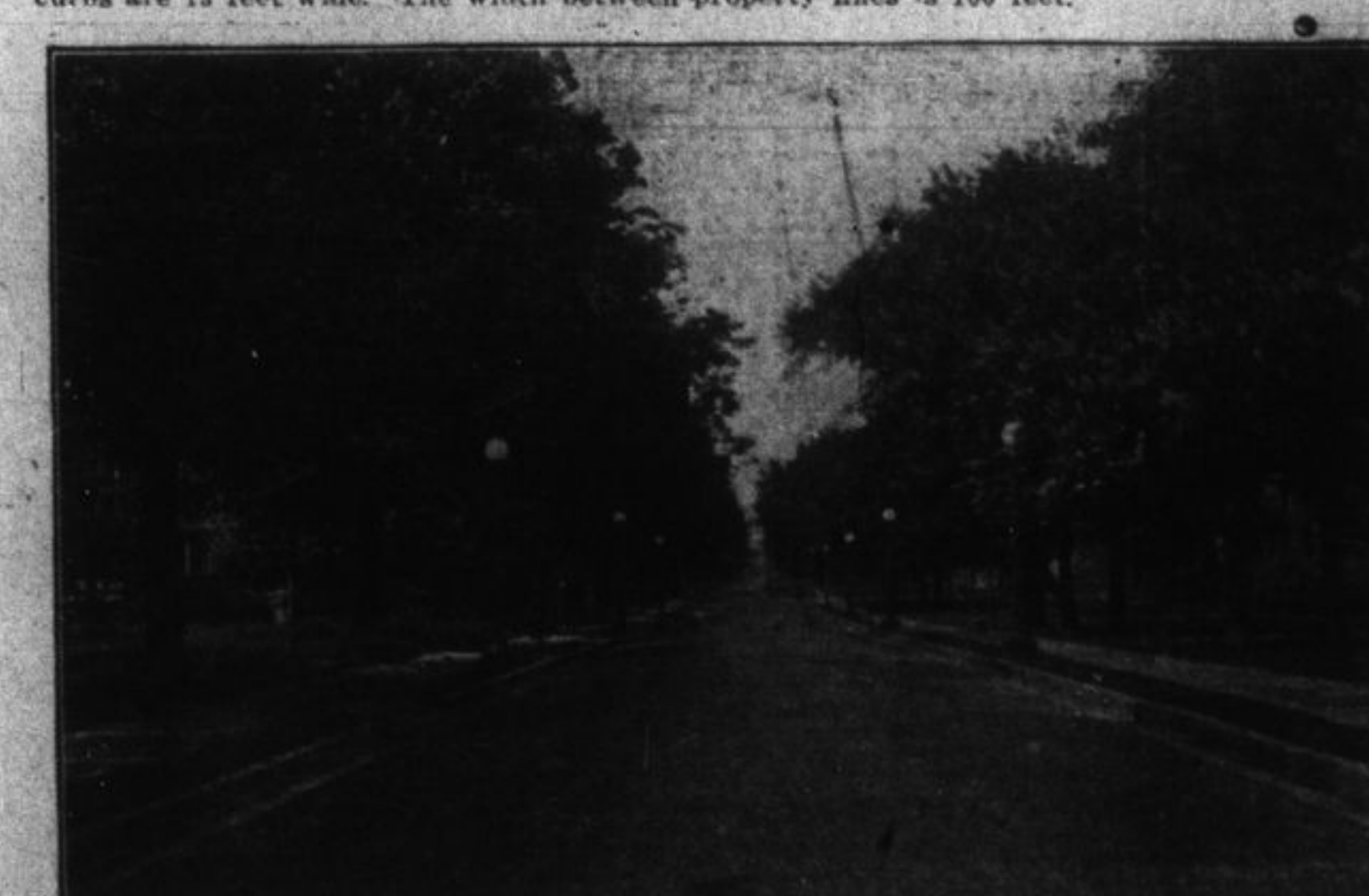
QUEEN STREET NORTH, KITCHENER. Bitulible surface 35 feet wide on a 5-inch concrete foundation, laid in 1912. The sidewalks are 5 feet wide and the grass spaces adjacent to the curbs are 3 feet wide.
