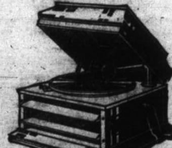
The instrument at the right is the \$50 Columbia Grafonola. It has the hinged enclosing lid, the tone-control leaves at the front, the new and wonderful Columbia reproducer and the powerful motor that plays three records with a single windin
