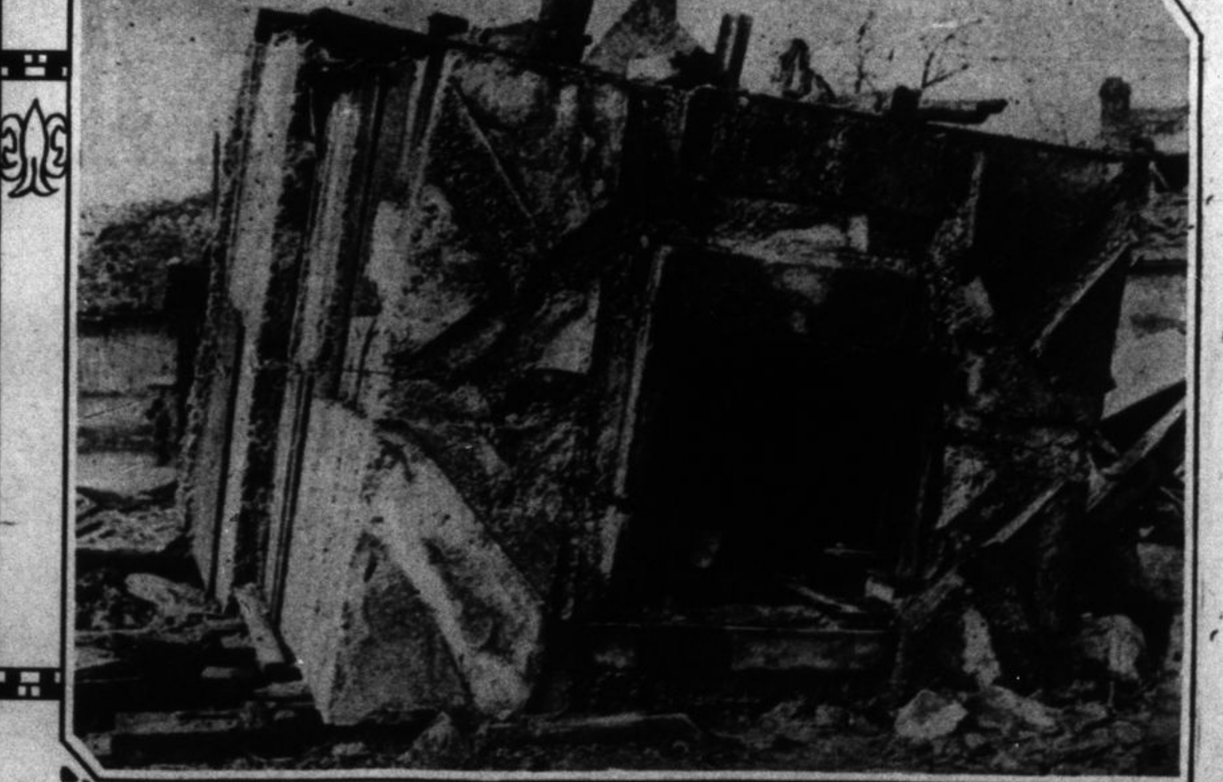
Type of German shelter, built of solid concrete, used by a machine-gun squad. The position of which it formed part was destroyed by the French mines, but despite the force of the explosion the shelter remained intact, though turned upside down. It is fortifications of this kind that give the famous Hindenburg line its so-called impregnable character.
