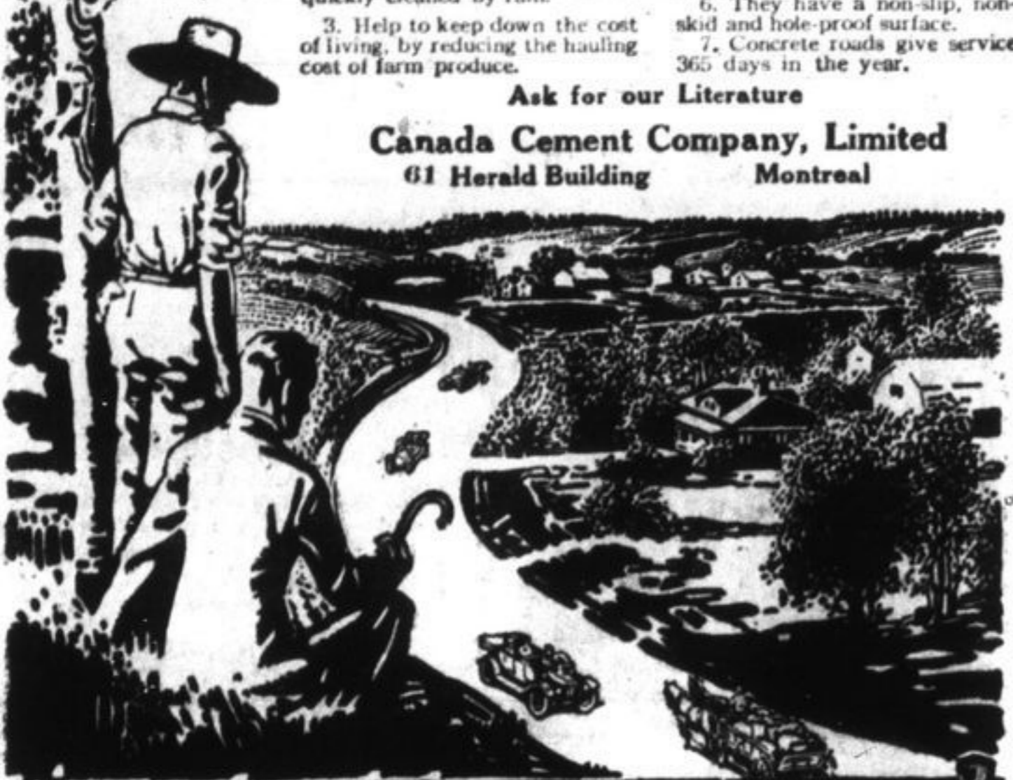
Concrete for Permanence
