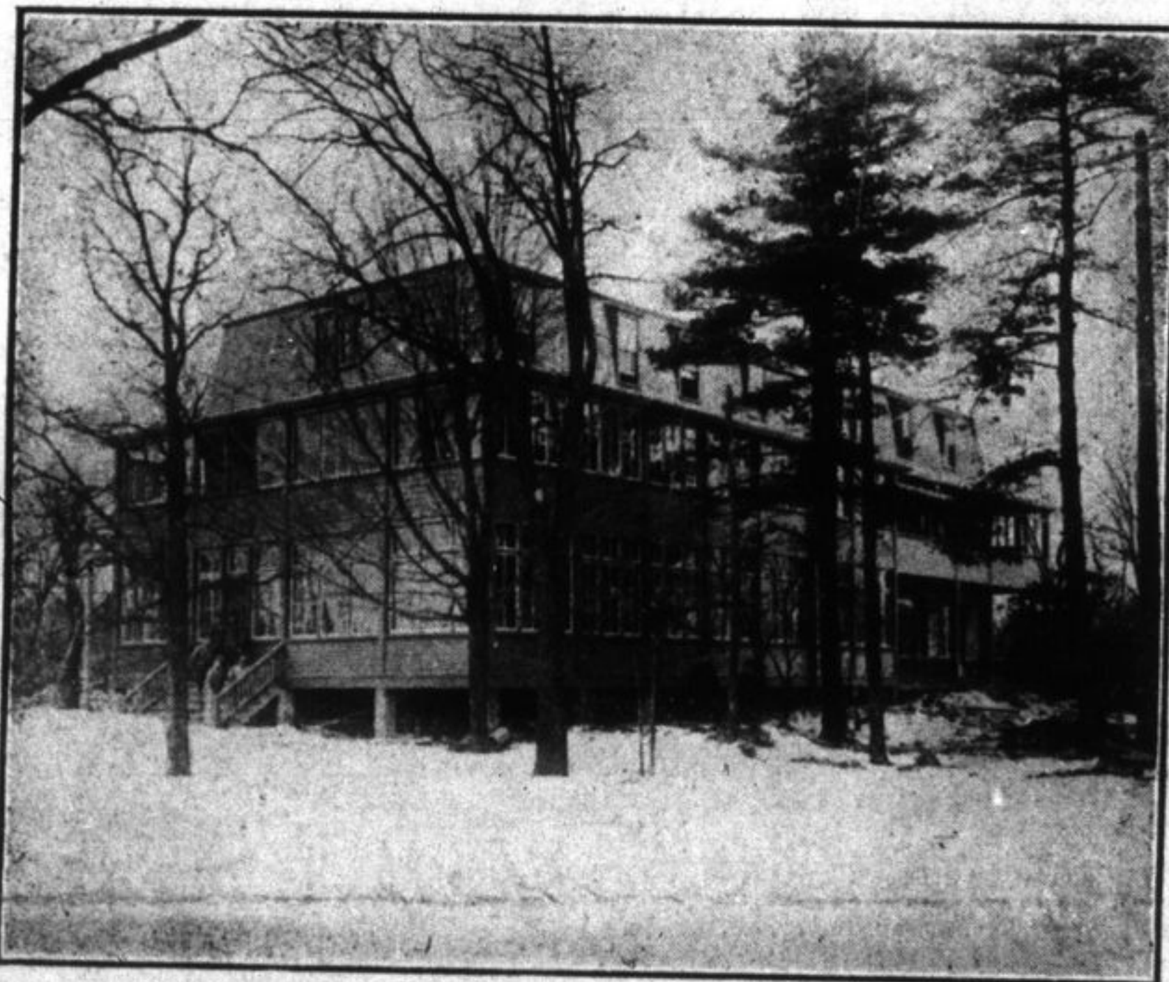
Alterations that have been made to the Staubenzie residence in the grounds of the Mowat Memorial Hospital.
