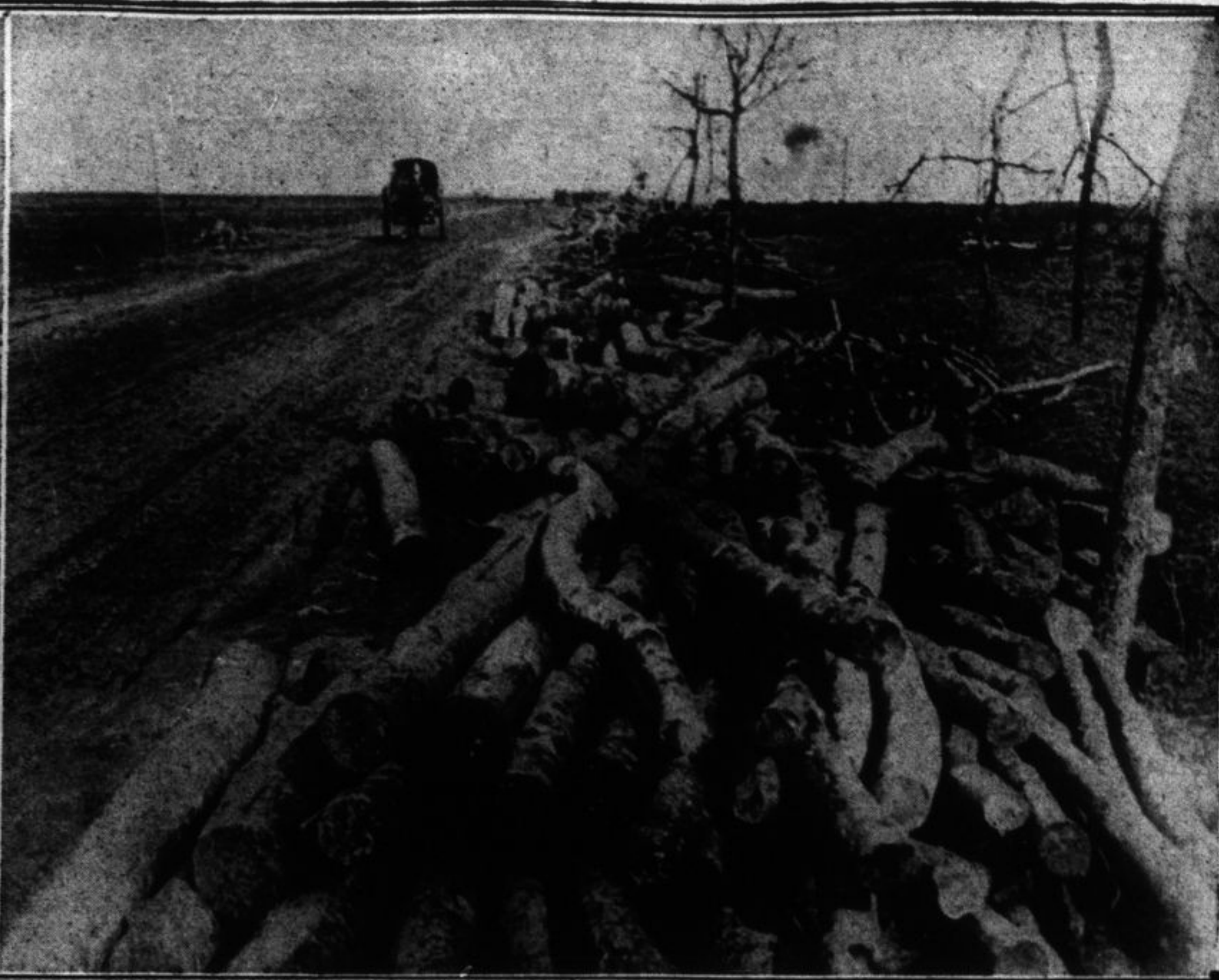
Winter will play havoc with the military roads in France which have already been torn up by shell fire, retarding the moving of guns and men. Forests will be denuded to supply the necessary wood to repair these. Photograph shows lumber made available by engineers.
