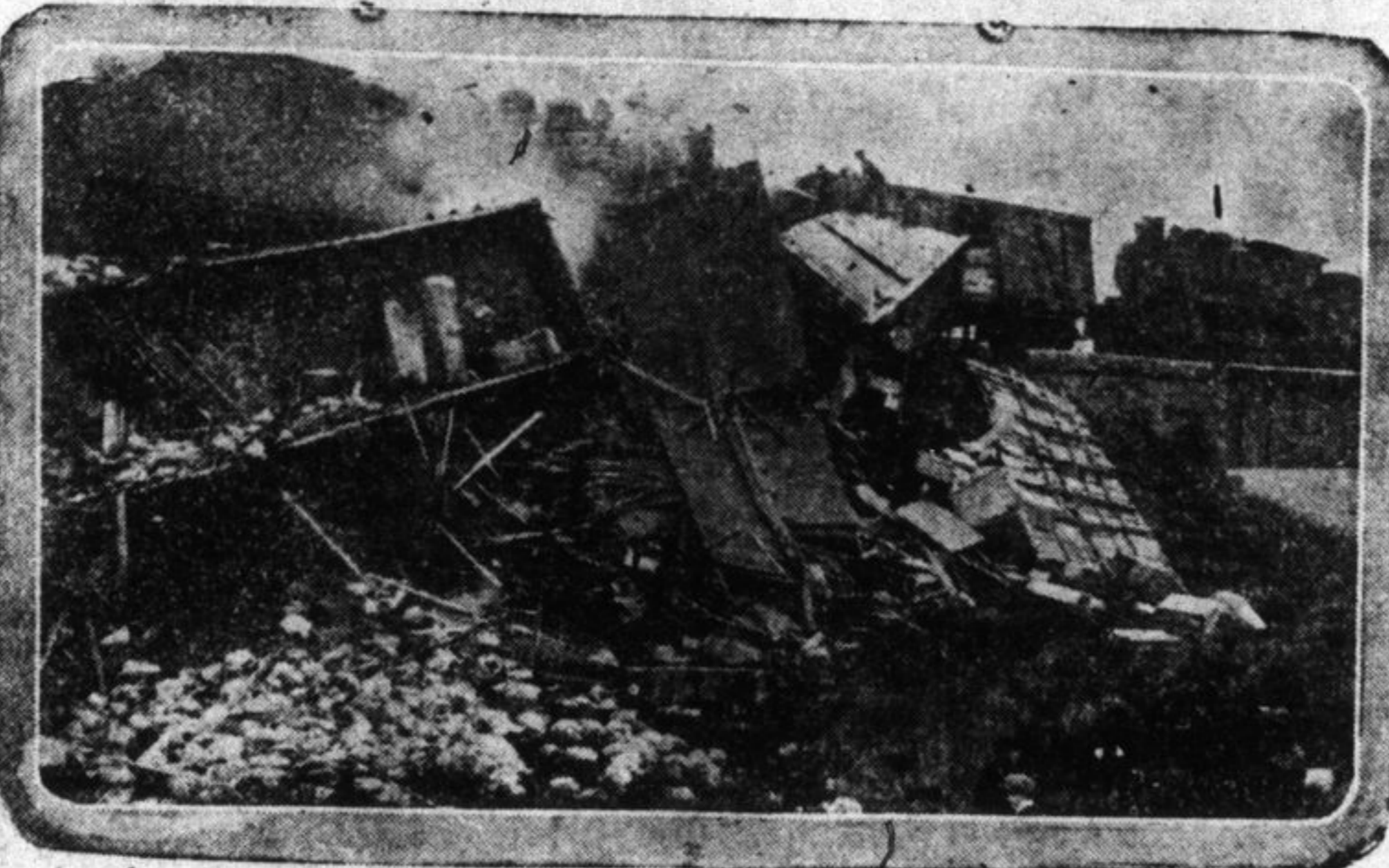
This unique picture shows wreck at the west end of the C. P. R. bridge at Gait, Ontario, in which six cars were reduced to matchwood, and Engineer Joe Brand, of Toronto, and Fireman Kusel, of London, saved themselves by jumping. The smash-up occurred on the main line and delayed traffic greatly. Slippery rails was given as the cause. The same spot was the scene of a bad wreck several years ago, when five men lost their lives. The white articles in the foreground are not mushrooms, but fresh hams.
