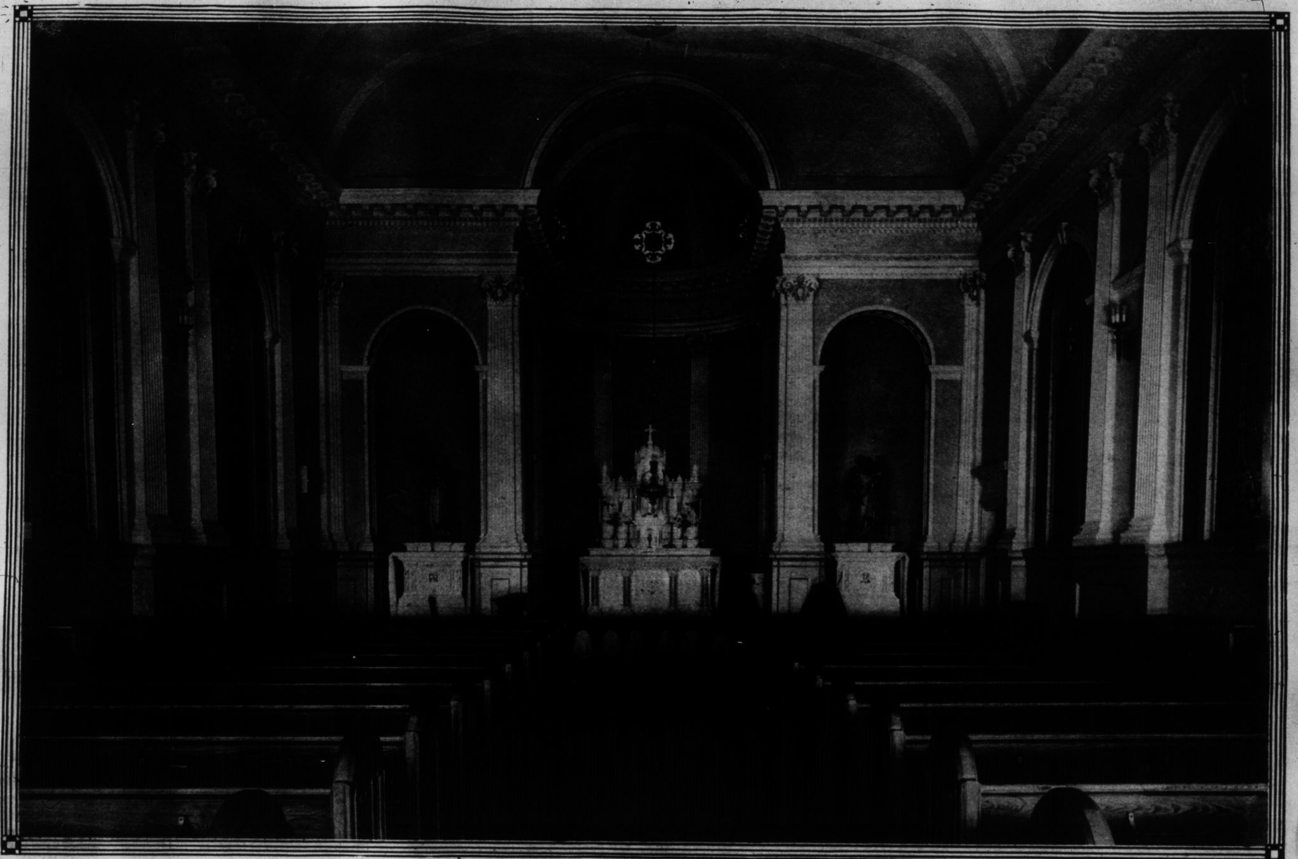
BEAUTIFUL NEW CHAPEL OF ST. JOSEPH'S HOSPITAL, LONDON, ONT. This handsome chapel is in the new wing of the St. Joseph's Hospital, recently consecrated by Right Rev. Michael Fallon, Bishop of the Roman Catholic Diocese of London. The hospital addition is one of the best equipped in the province, and the chapel is in keeping with the remainder of the building.
