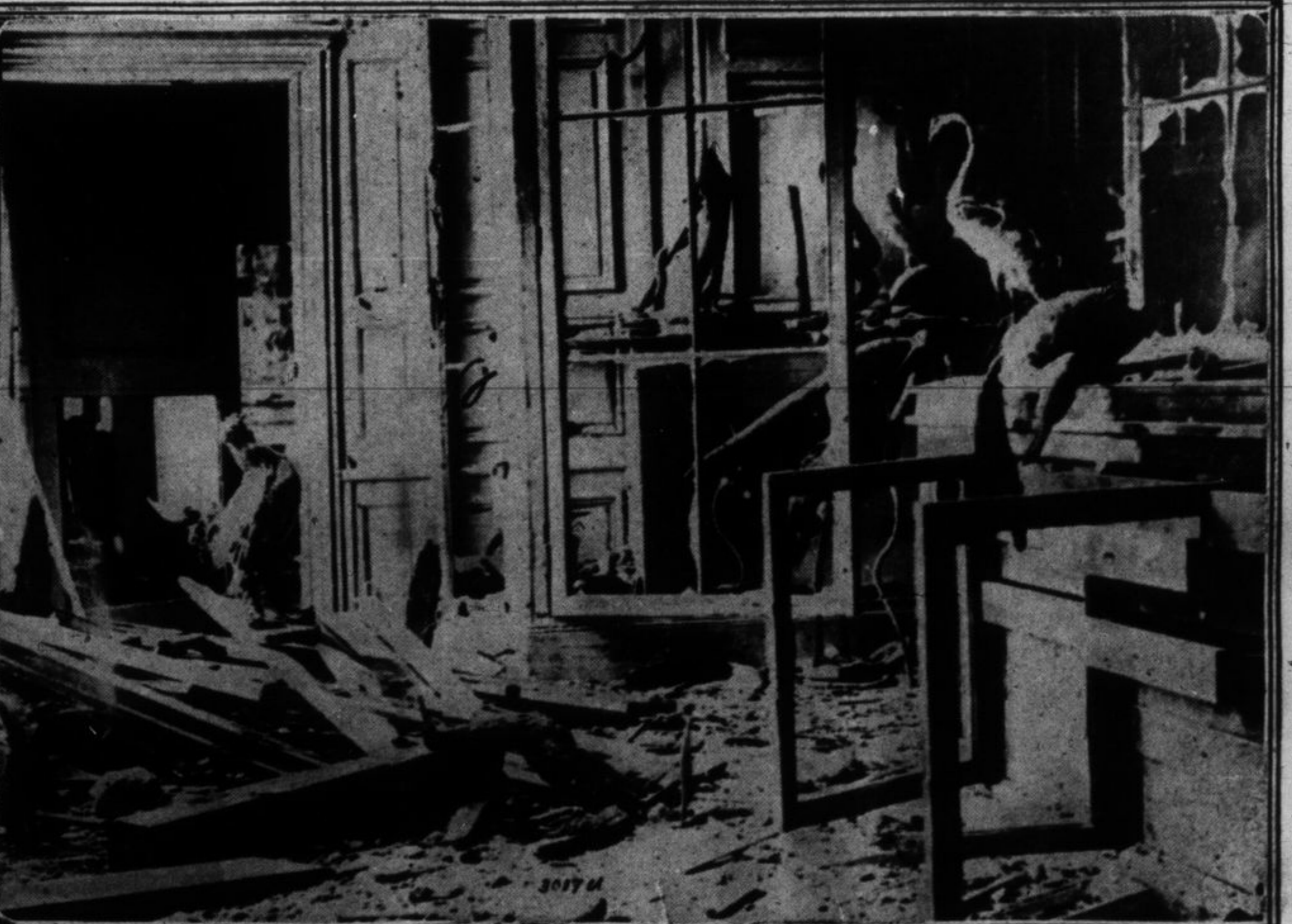
HISTORIC MUSEUM DESTROYED. The interior of the Natural History Museum in the destroyed city of Verdun, showing all the stuffed animals knocked to pieces by the German shells.
