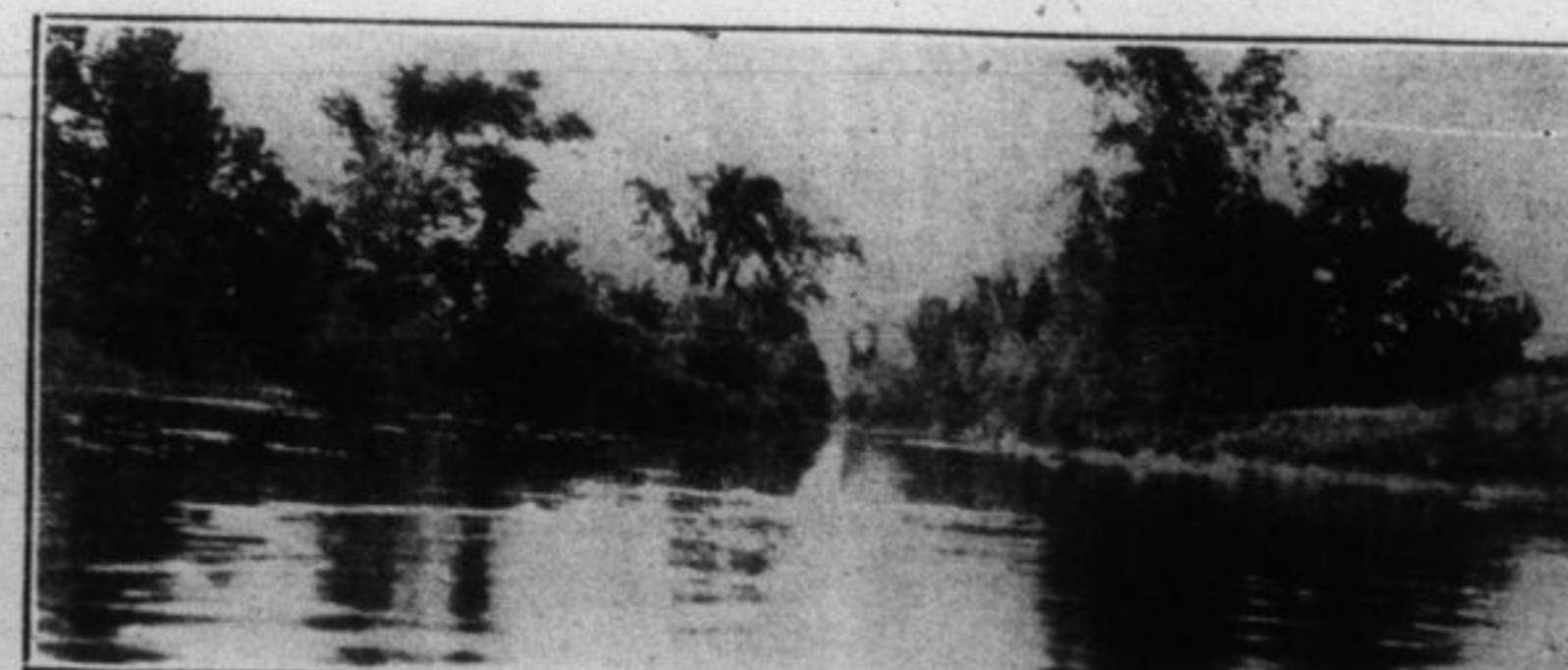
VIEW OF NAPANEE RIVER ABOVE THE FALLS.
