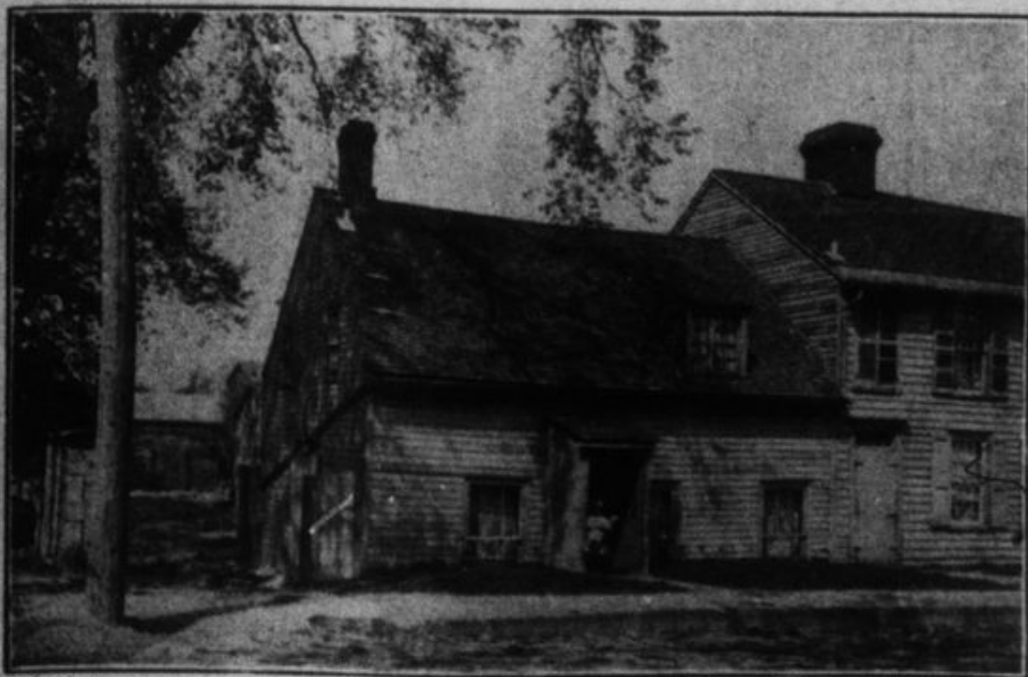
"GOVERNMENT HOUSE," KINGSTON, ONT. Where Col. John Graves Simcoe met his Executive Council, July 17th, 1792, and took the necessary preliminary steps to the opening of the first Parliament of Upper Canada.
