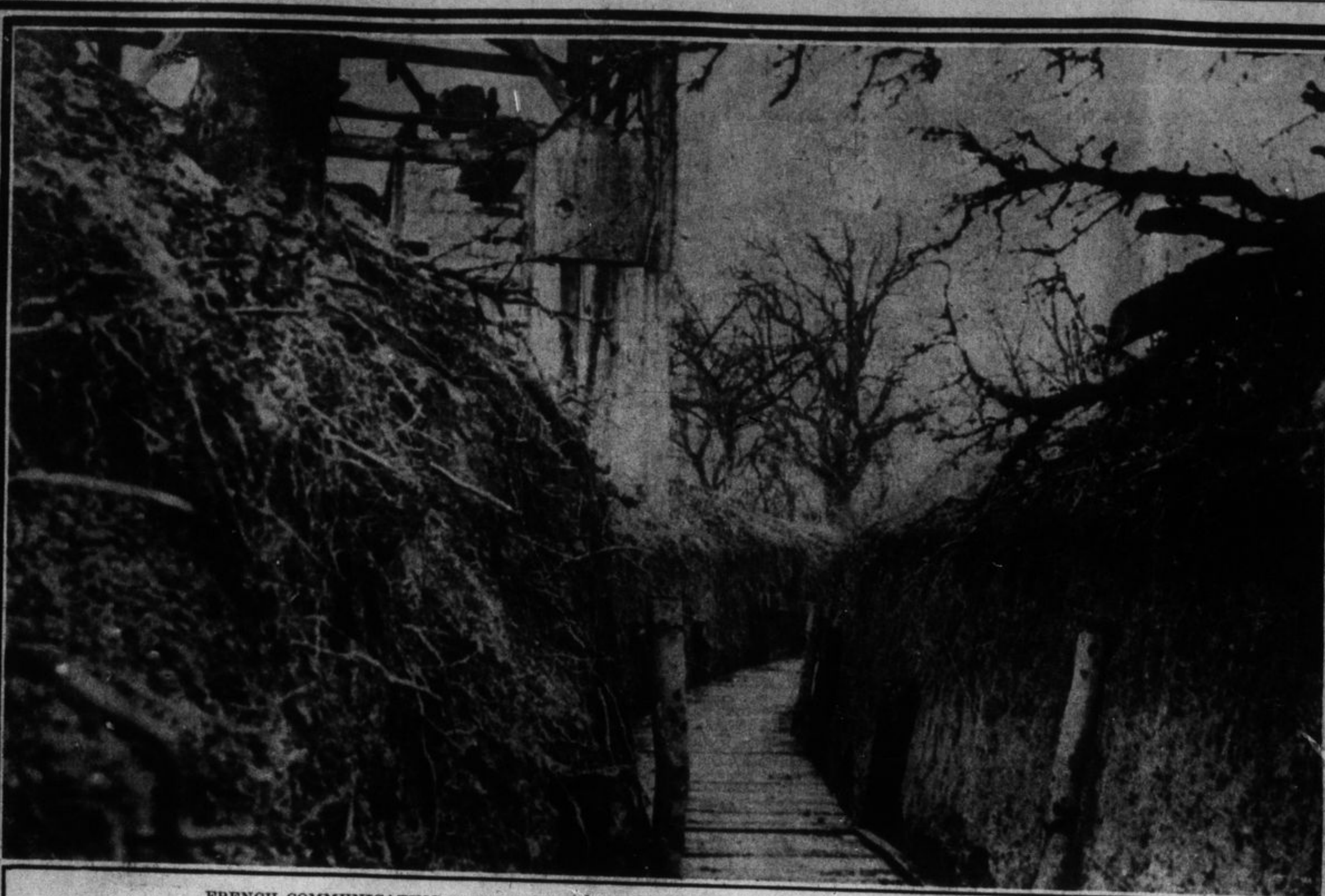
FRENCH COMMUNICATING TRENCH FILLED WITH WATER, BRIDGED TO PERMIT PASSING OF SOLDIERS. This is a French communicating trench, which was filled with water almost waist high. In order to permit of its use it was necessary to erect a bridge of boards for almost its entire length.
