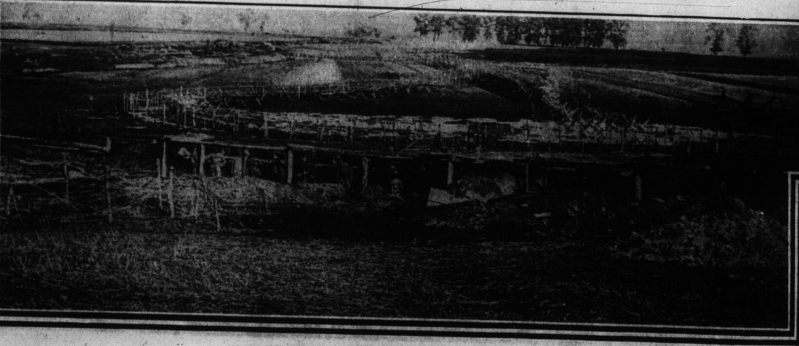
AUSTRIAN INFANTRY TRENCHES IN A SWAMP. Trenches of an Austrian infantry regiment in a swamp. The trenches have been built on top of the ground instead of dug in because of the fact that water was found a few inches below the surface.
