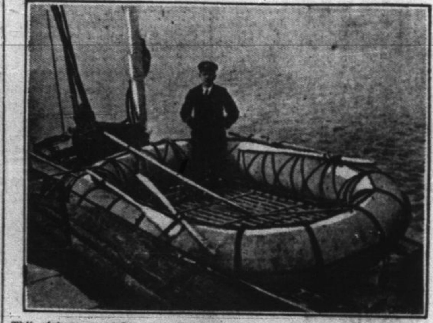
This picture was taken on a light cruiser and shows a large-sized Calley life-buoy, which will sustain forty-five persons. The space within the buoy is filled with wood-grating and the buoy is supplied with paddles. This valuable life-saving device has just been supplied to the ships of the Royal navy.
