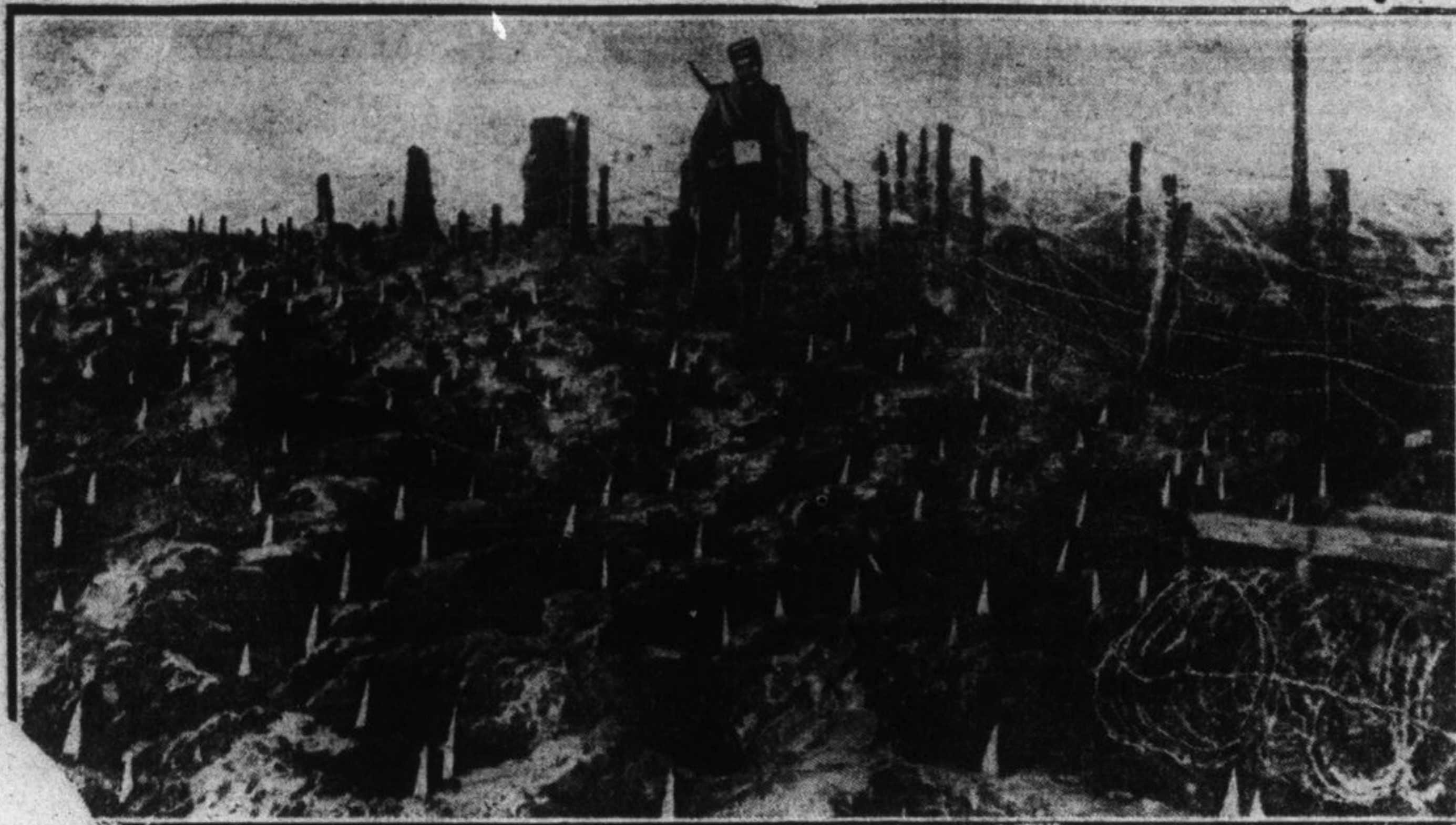
AUSTRIAN ENTANGLEMENTS TO IMPEDE ENEMY. The picture shows the pitfalls, surrounded by sharp spikes which the Austrians construct near their fortresses. The barbed wire on the right of the picture is heavily charged with electricity which would prevent any number of soldiers from gaining access to the fortress even though they succeeded in passing the pitfalls.
