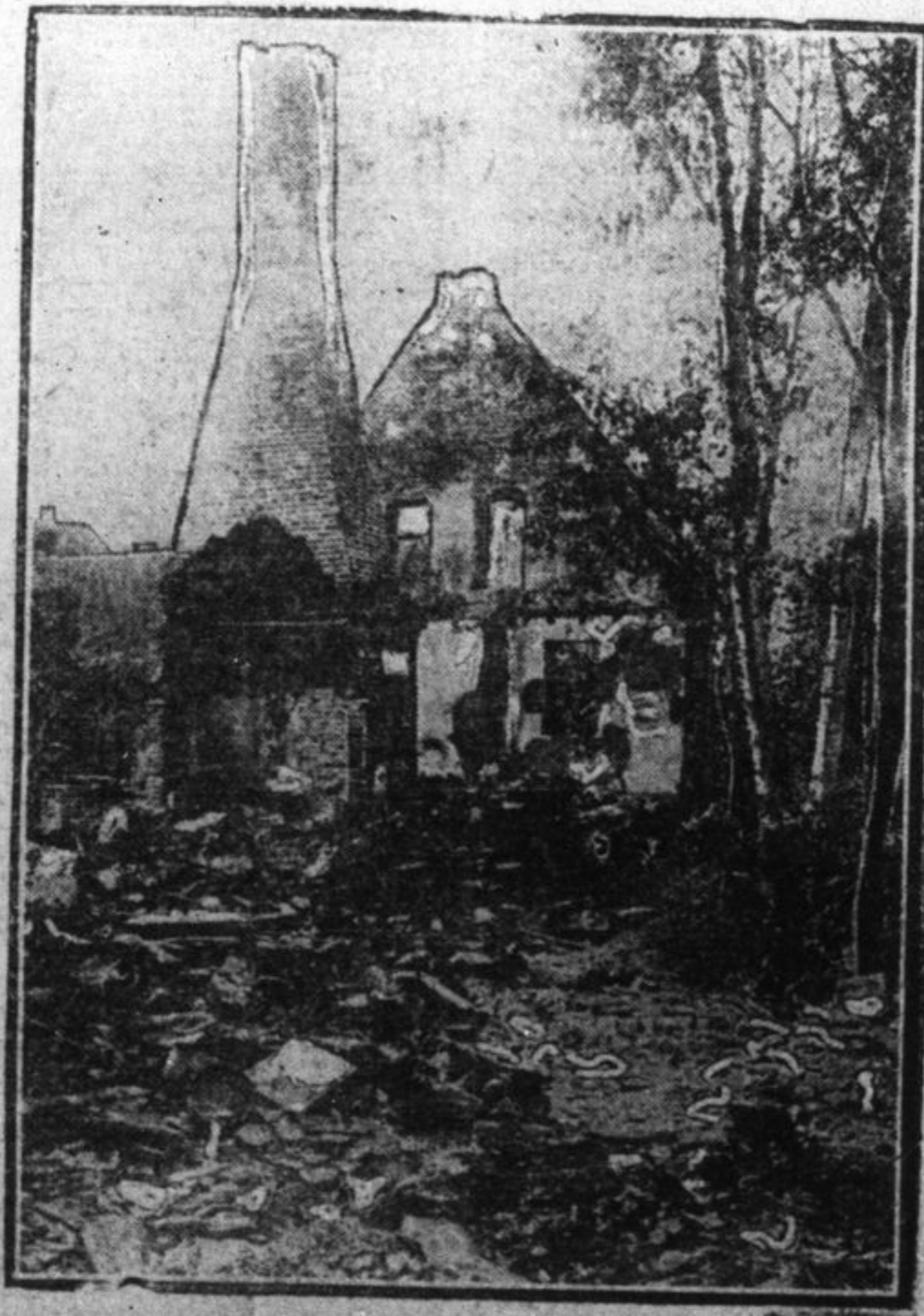
IN THE PATH OF THE DEVASTATING GERMAN ARMY. Ruins caused by German artillery fire at Boore, France.
