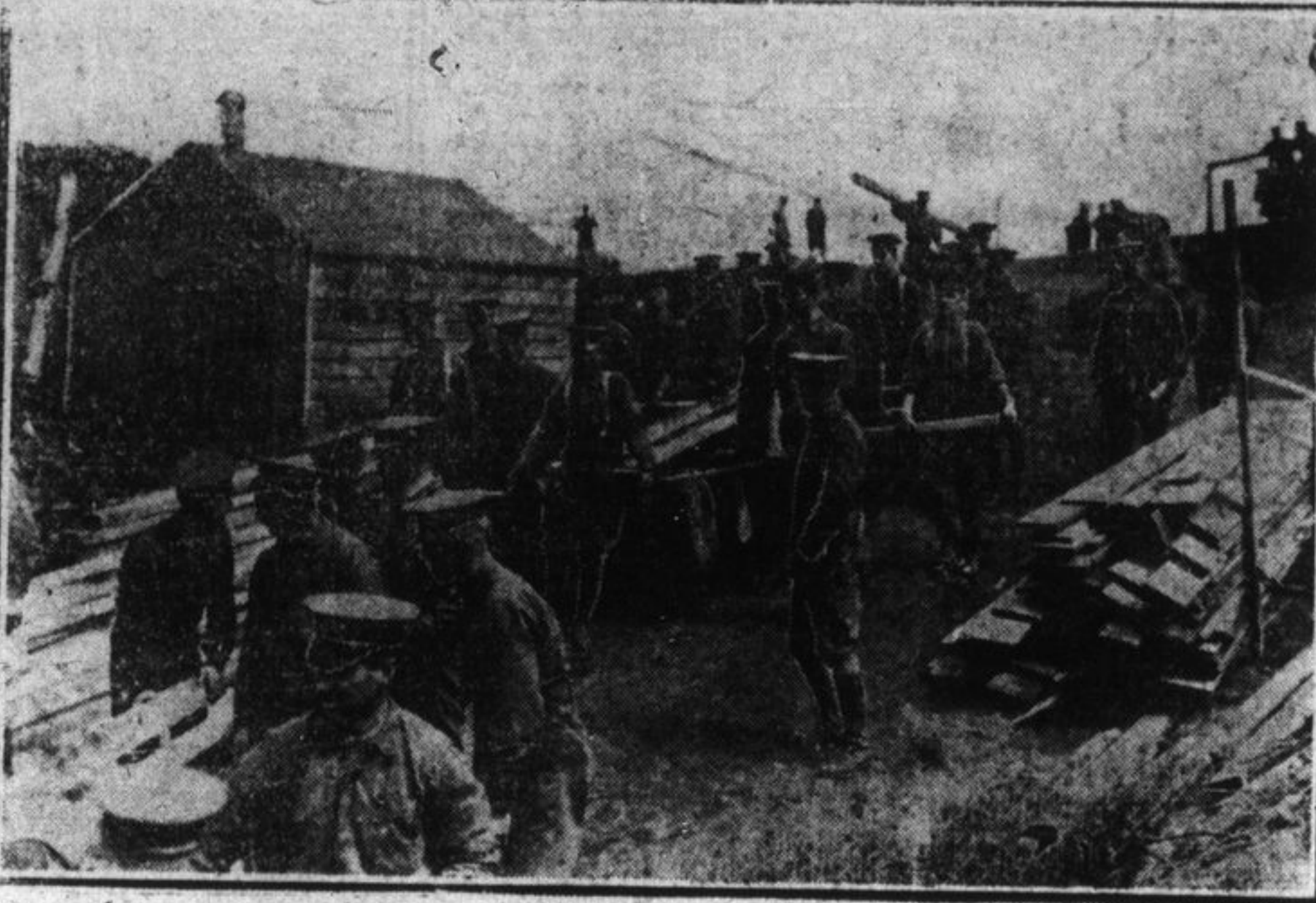
300 ROYAL CANADIAN ENGINEERS BUILDING PONTOON AT CAMP.
