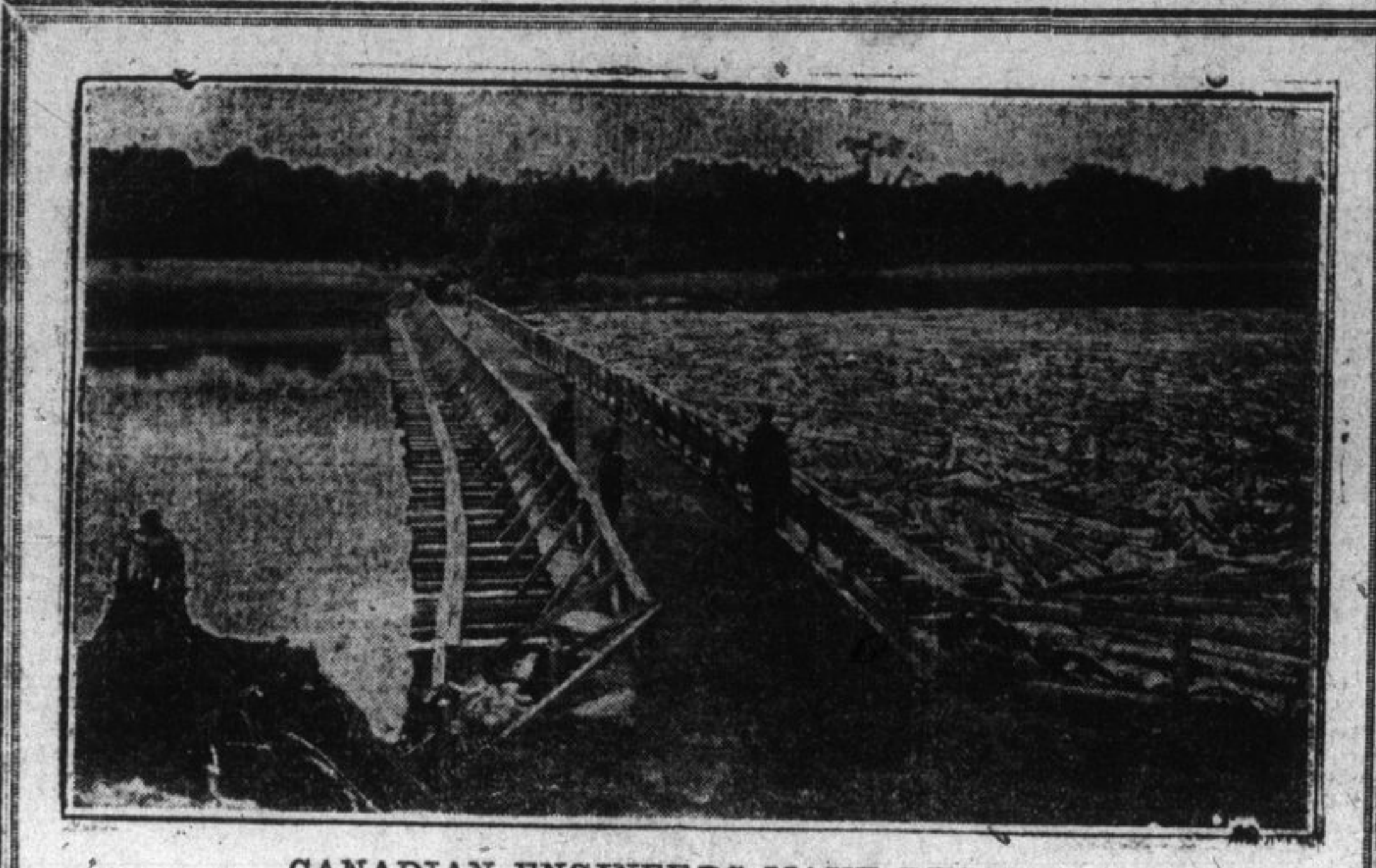
CANADIAN ENGINEERS MAKE RECORD. An artillery pontoon, three hundred and fifty feet long, over the Jacques Cartier river, which was built by three hundred men of the Canadian Engineers in four hours. This is a record for this type of pontoon.
