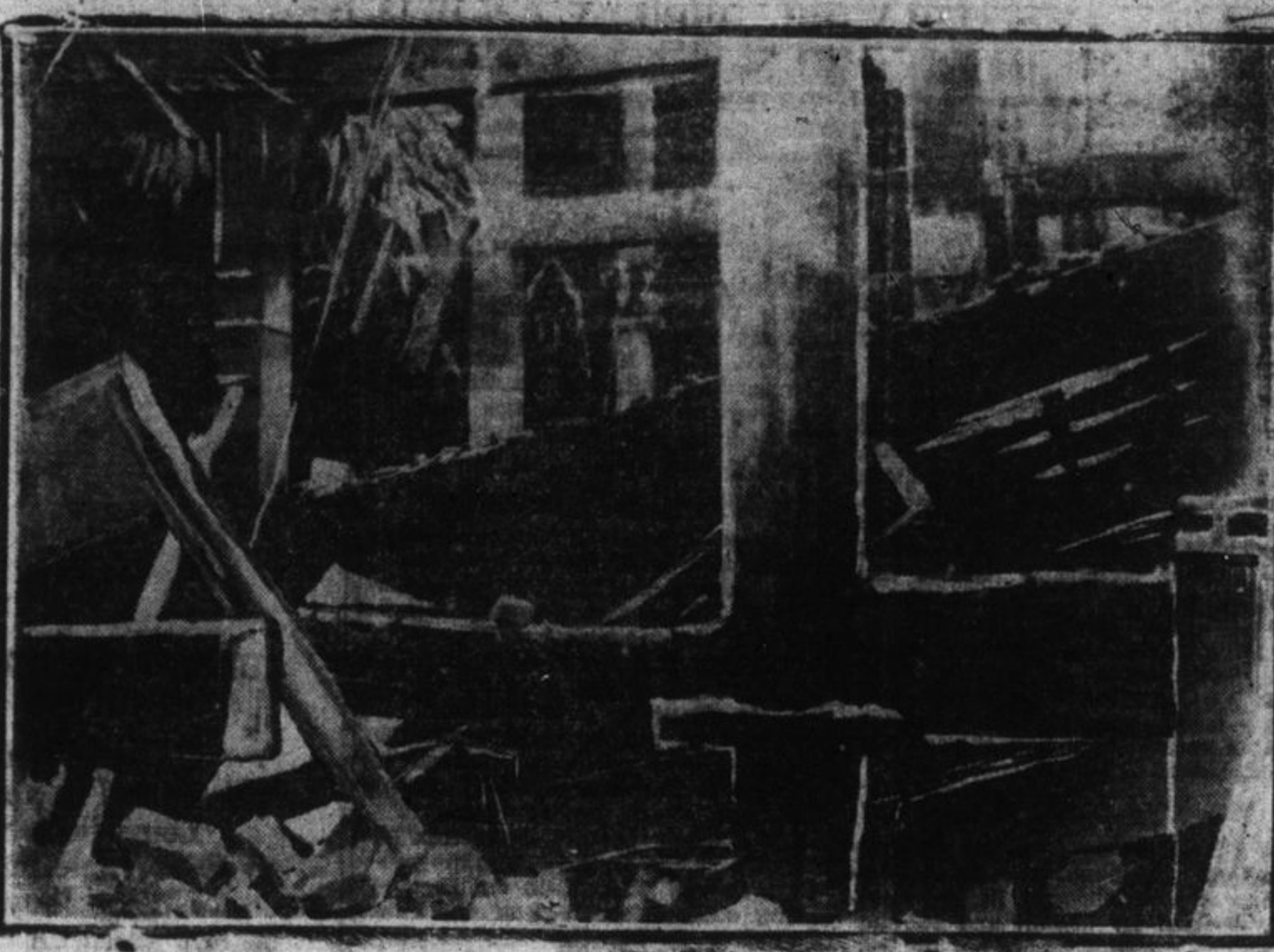
TORONTO'S FALLING WALL CATASTROPHE. The above picture shows where the bodies of Sadersky and Cohen were taken from the ruins of the wall of the Independent Cloak Company, the ruins of which, after being gutted by fire last January, were left standing. By instructions from the City Architect, Albert Strong, an expert wrecker, was given the job of demolishing the building, shortly after the fire. When the building was in a safe condition, it was turned over to Weinerman, the owner of the building, and also a wrecker. He discharged Strong and employed a number of foreigners. The men were poorly paid, and totally ignorant of their work, and this is held responsible for the collapse. Two killed and six injured is the toll of the disaster.
