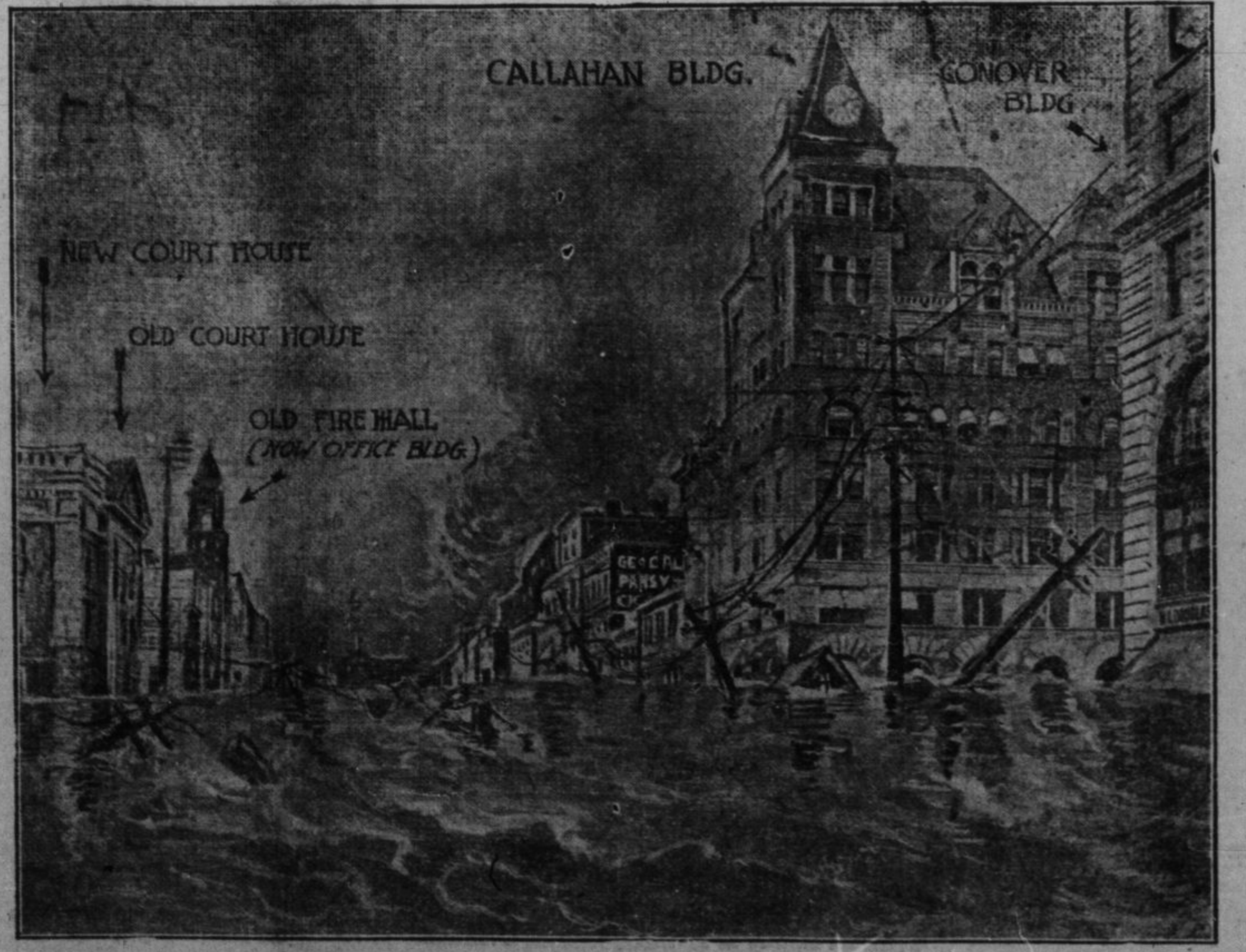
SHOWING THE CHIEF BUILDINGS AND INDICATING THE RUSHING WATERS WHEN THE FLOOD WAS AT ITS HEIGHT.
