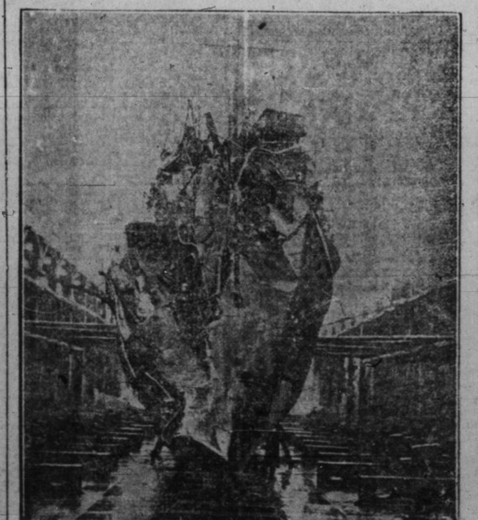
CRUMPLED BOWS WHICH WERE SET STRAIGHT WITHIN TWENTY DAYS.
