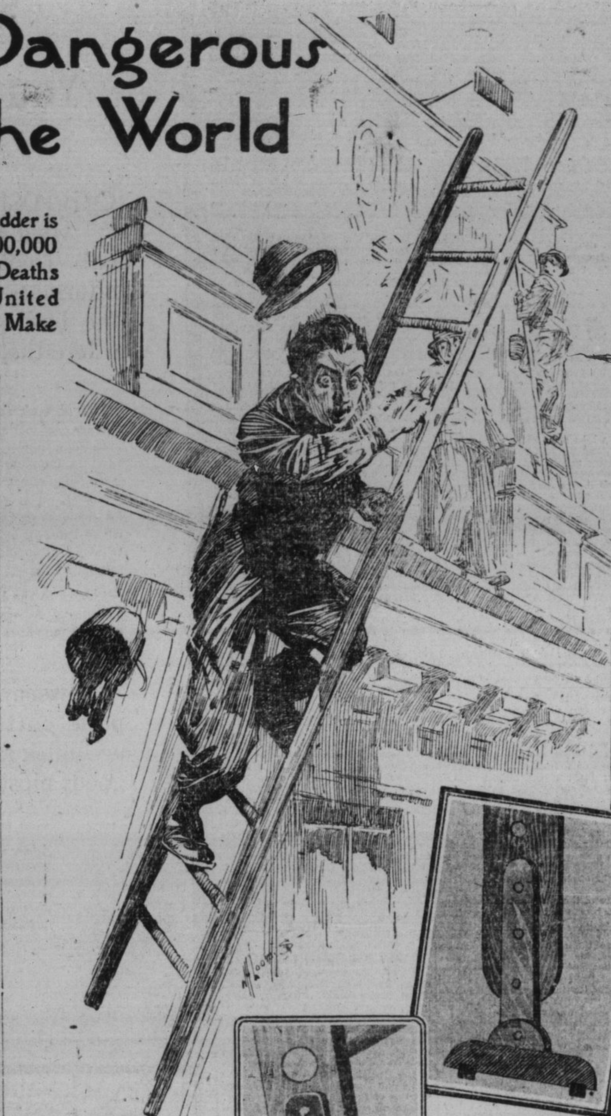
Ingenious Practical Safety Shoe for Ladder Feet German Origin. A Heavy Rubber Ring, Set in Wooden Shoe, Has the Advantage of Section as Well as Friction.
